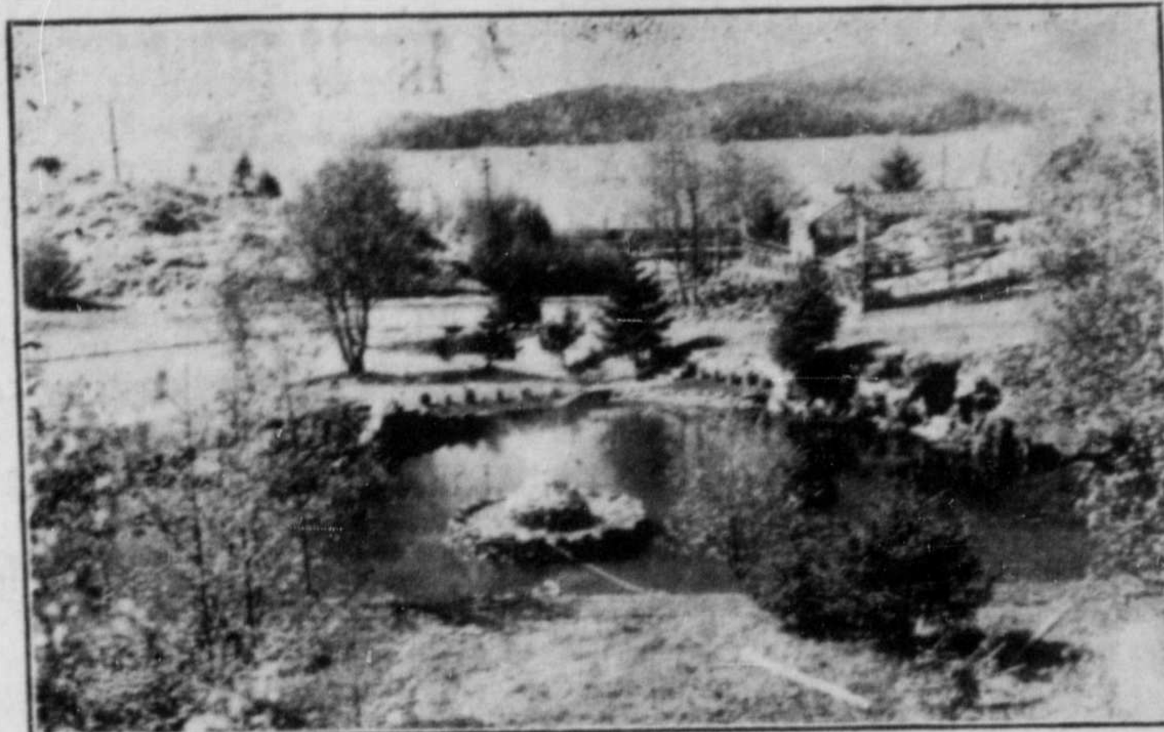
Picturesque pond converted by Canadian National Railways from dirty excavation hole.
