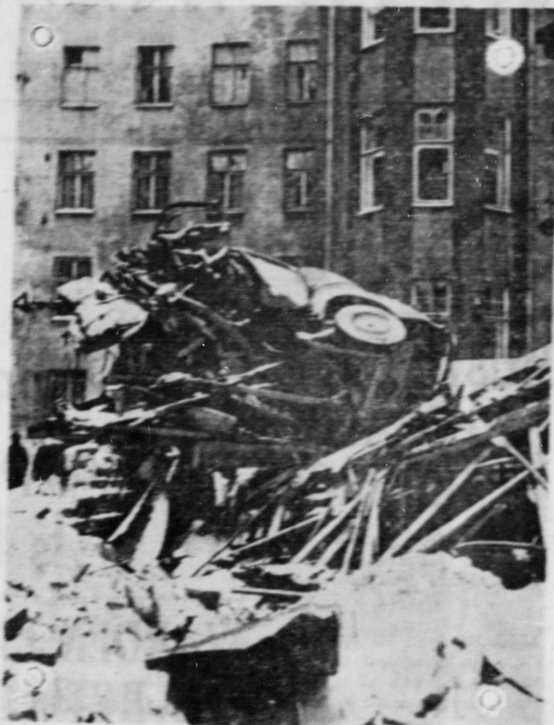
Street scene in a Finnish town showing scope of the debris piled up from a Soviet demolition bomb's direct hit. Part of an automobile is on top of the wreckage of a house.
