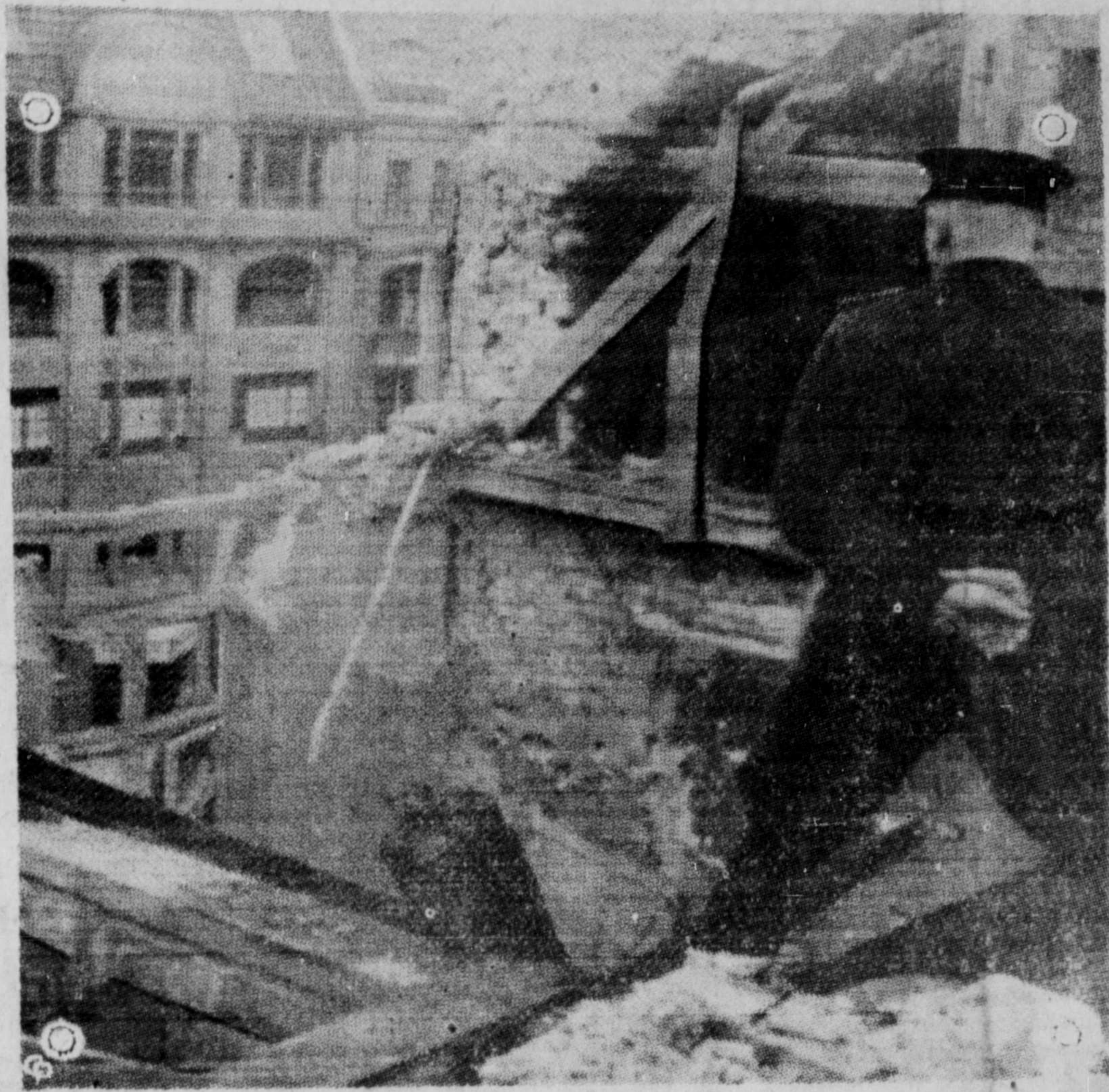
A German fireman looks into the wreckage of a building on Kottbuser Strasse, Berlin, less than two miles from Wilhelmstrasse, where German government buildings are located. This building and others in the vicinity were bombed by British airmen retaliating for German bombings of London.
