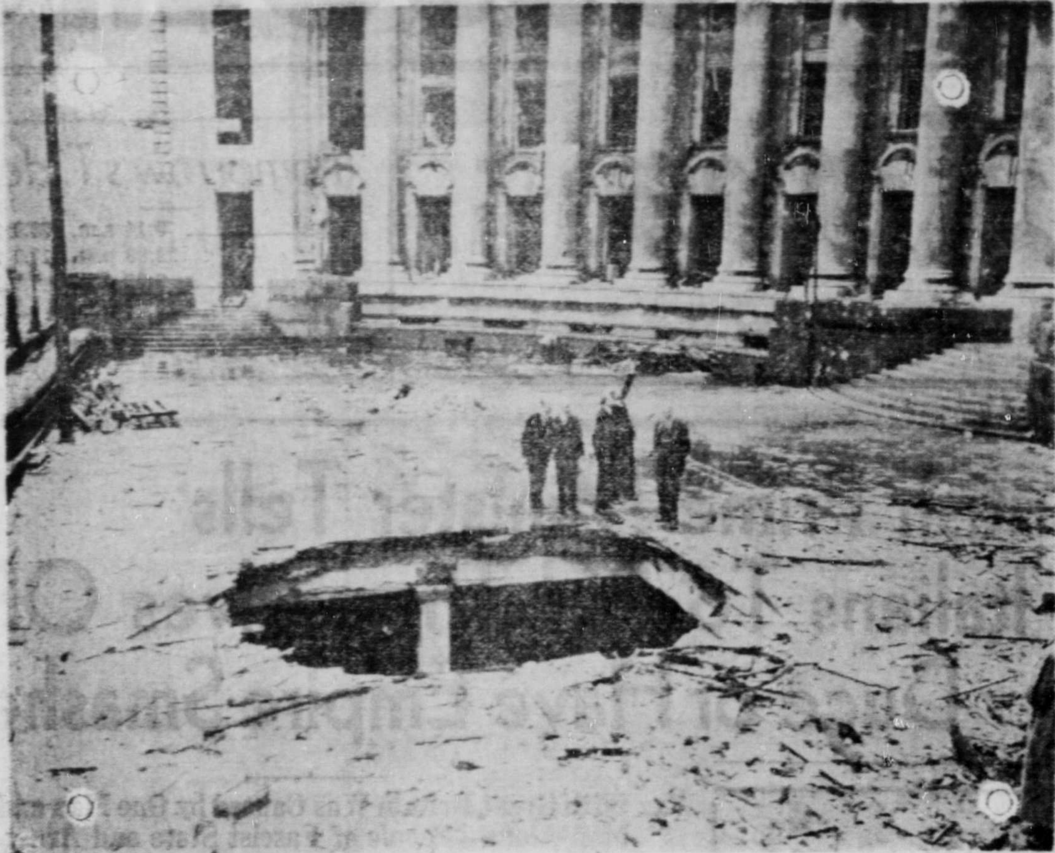
The huge crater was torn in the pavement outside London's county hall during the air raid of September 19. The bombs went clear through to the cellar before exploding.
