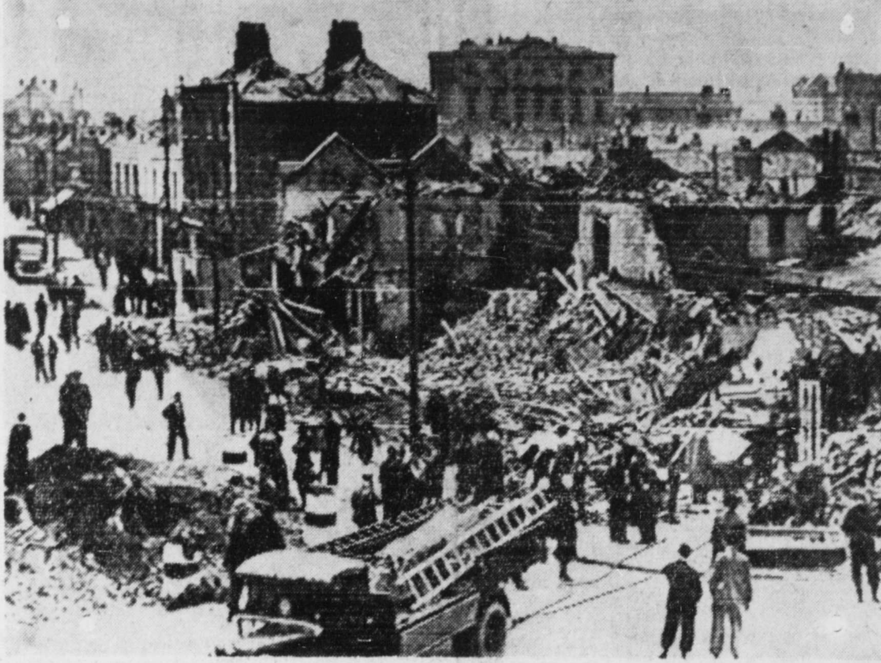
This scene in the North Strand, one of the main business sections of Dublin, shows the severe damage done by an air raid from unidentified planes. Rescue squads found more than 30 slain, 25 missing and 300 injured in the May 31st bombing of the Eire capital. After examining bomb fragments, Dublin blamed Germany for the raid. This was the second raid on Dublin and the ninth on the country. Eire is nominally neutral in this war.
