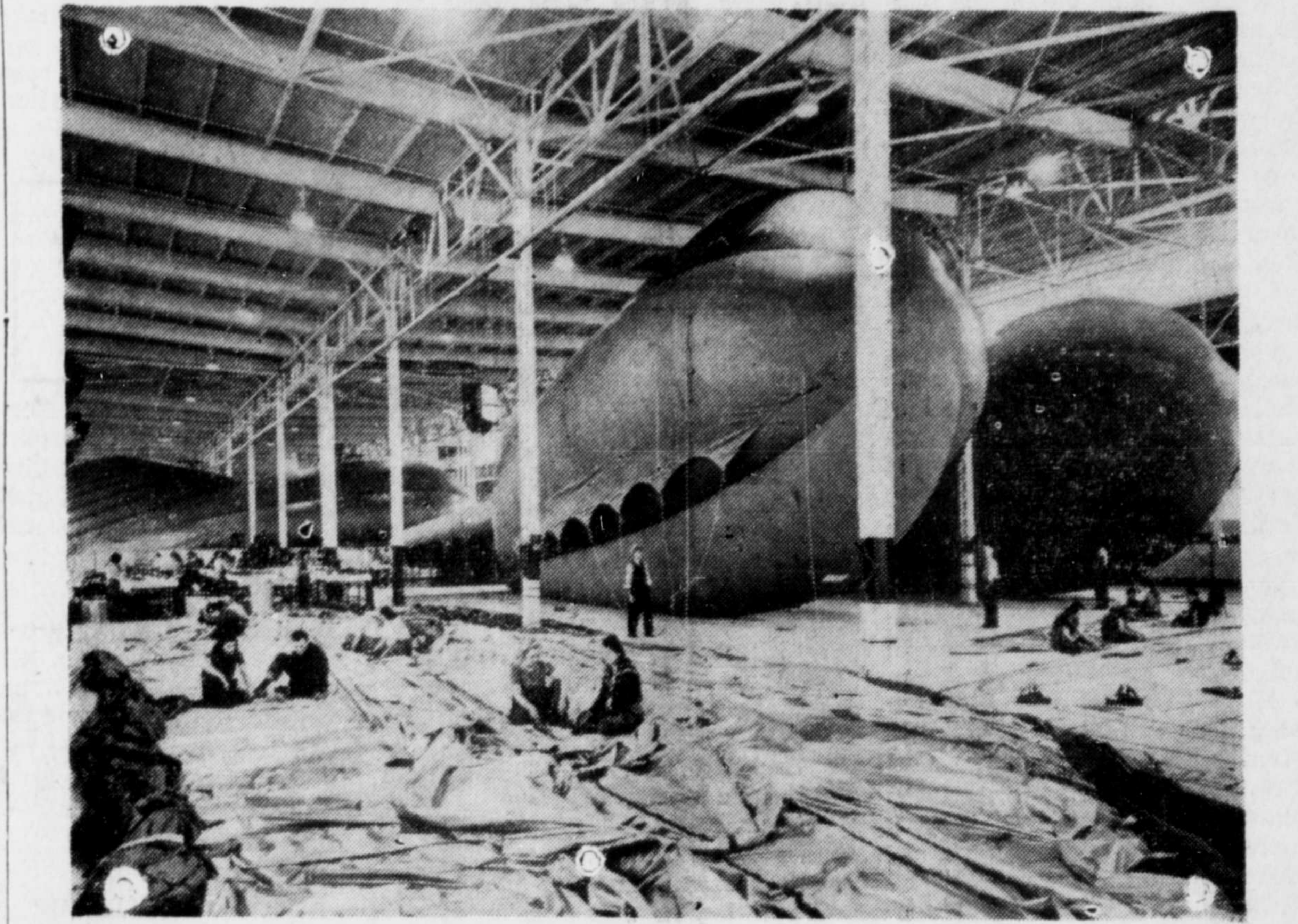
A view of the new huge balloon room at the plant of the Firestone Tire and Rubber Co. in Akron, O., where as many as 12 great barrage balloons may be inflated at one time.
