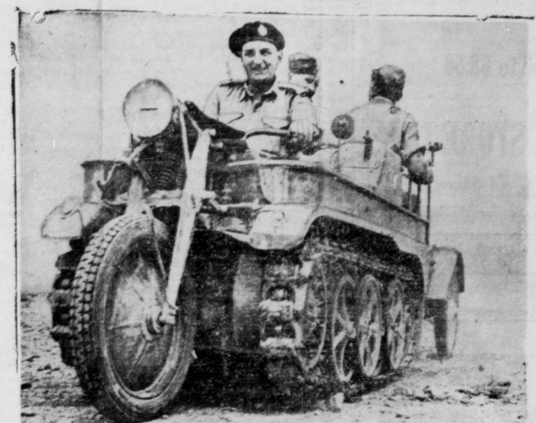
This strange gadget, hybrid motorcycle and tank, was one of the pieces of equipment captured by the British in the Libya-Egypt fighting. The vehicle is very manoeuverable and is used for carrying a few men or towing small guns at fairly high speed.
