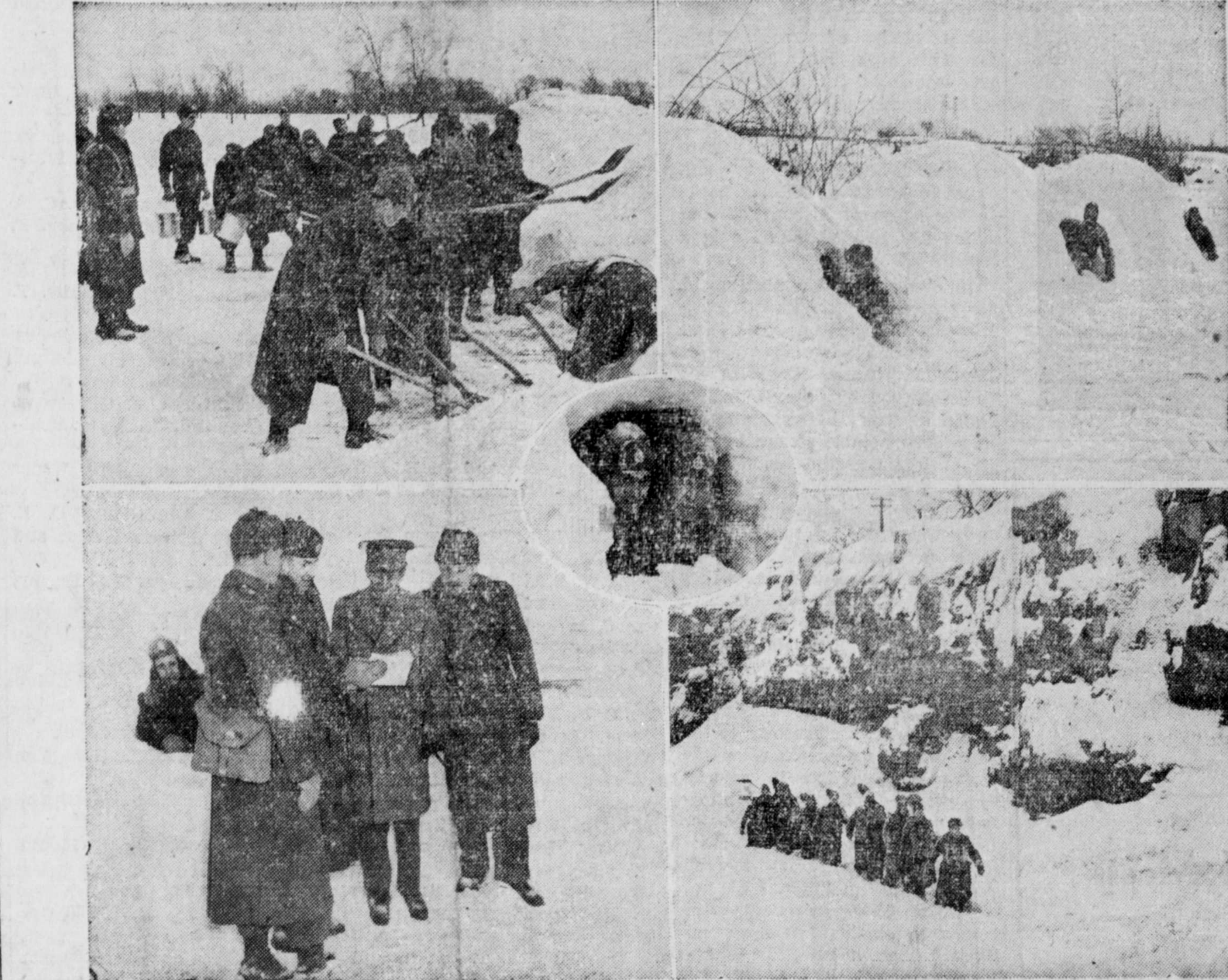
The Regiment de Maisonneuve (2nd Reserve Battalion) took the initiative in winter warfare manoeuvres in the 34th Reserve Brigade Group in Montreal this winter. Here they are pictured building intercommunication huts. Upper left a platoon of men start the first phase of building the huts. Pictured in the background are water carriers whose job it is to make the huts solidly packed with ice and snow. Upper right shows the huts finished and men in them. The purpose of the huts is to house advance scouts or field telephones to relay the enemy's forward positions. Lower left Col. Paul Grenier, Commanding Officer of the 34th Reserve Brigade, second from the right, views plans drawn up by Major Hughes Mitchell, second from the left. Two members of the Regiment de Maisonneuve are seen in the insert looking from their finished hut. Their job finished, a work party is seen in the lower right picture marching back to their base after a strenuous week-end.
