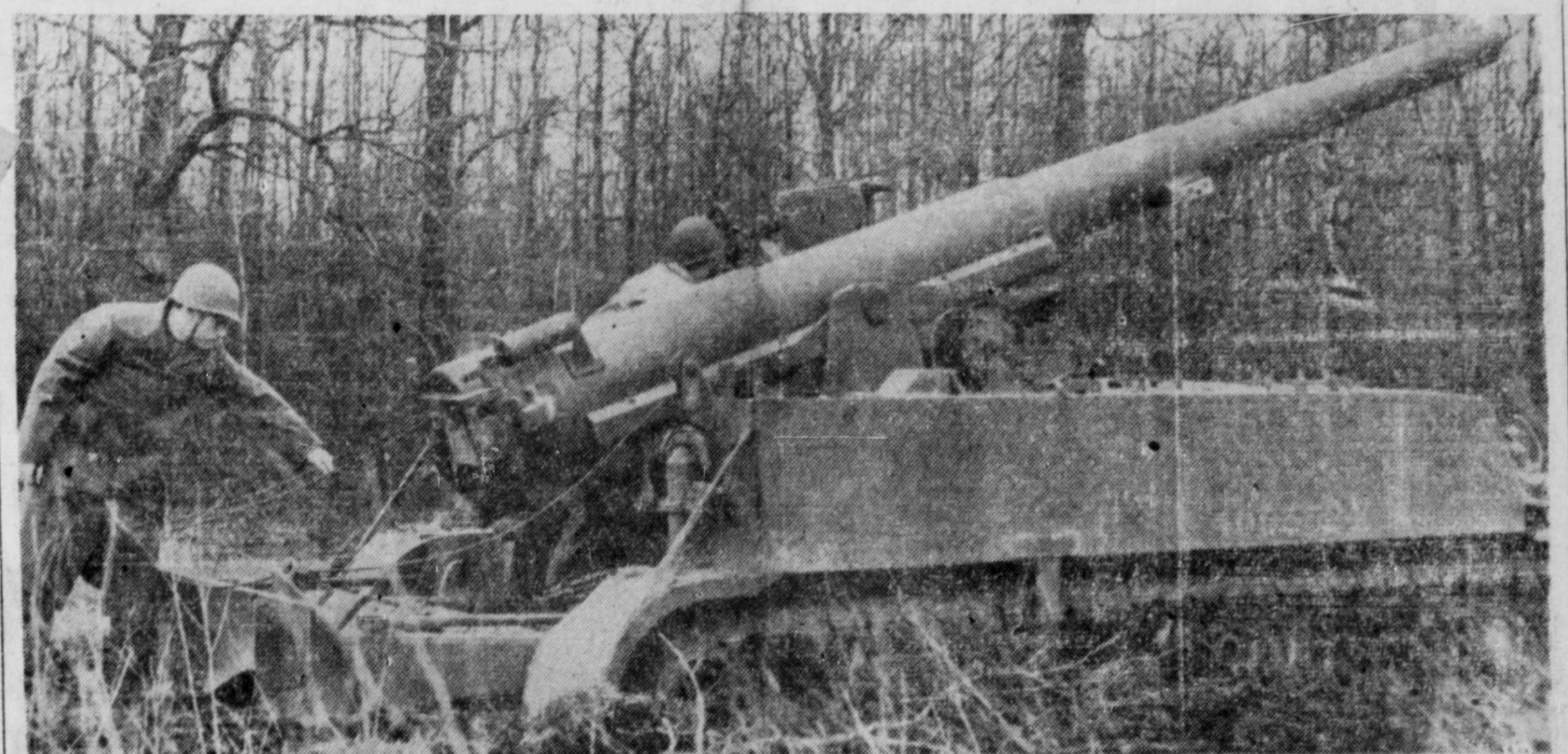
Here is the U.S. Army's new M12, described officially as a gun mounted gun-motor carriage and is said to be more than a match for any jectile more than 10 miles. It is also a highly mobile weapon, atof the tanks now being used by the enemy. Its 155mm. all-purpose taining the speed of a medium tank.
