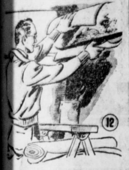
Renew Insulation we coal by trapping the in furnace and pipes. lace faulty insulation. ter and metal are such good t conductors that fuel will wasted unless these parts well insulated.
