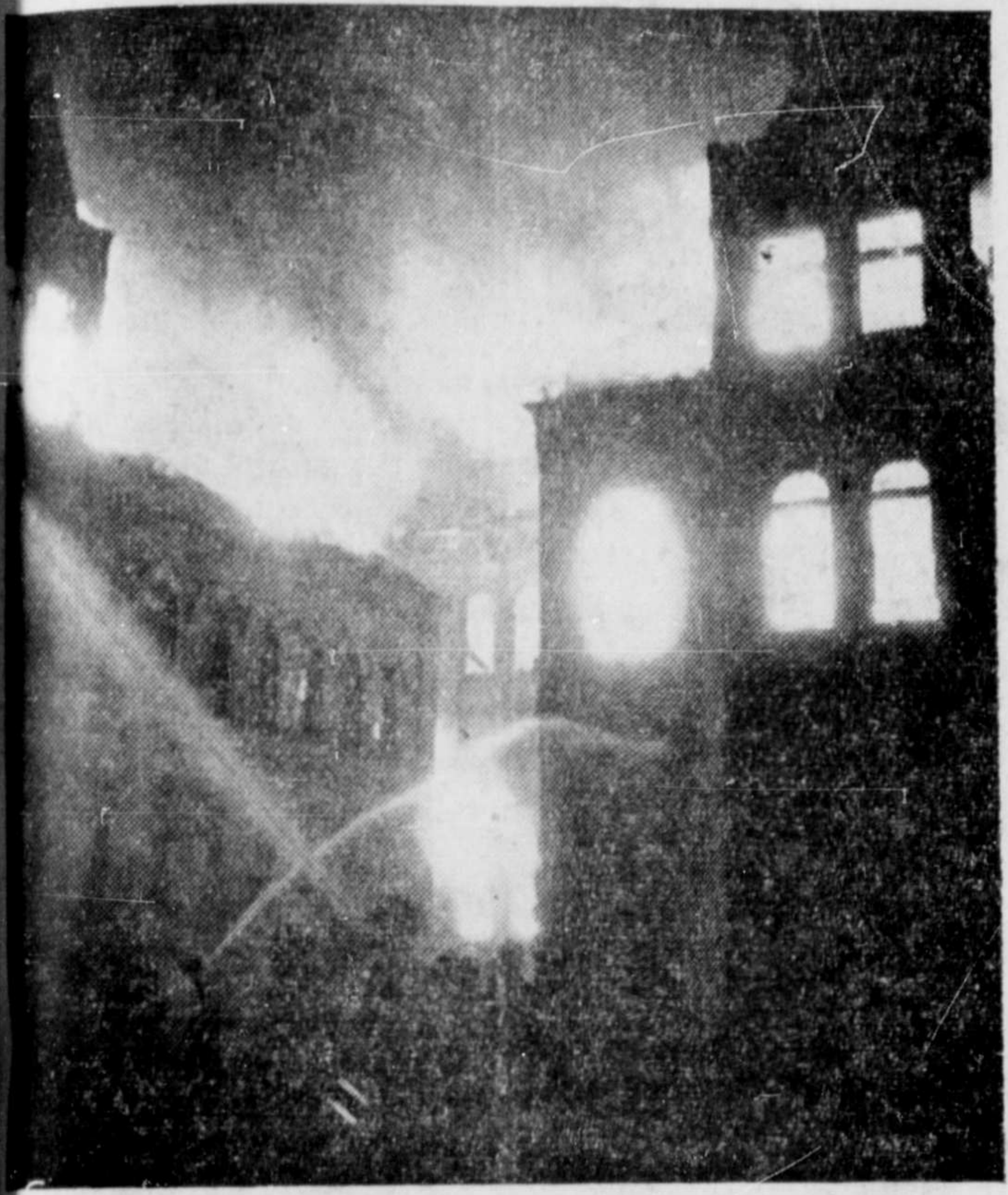
COLLEGIATE IN HAMILTON, ONT., DESTROYED—One of Ontario's oldest and most famous colleges, "Old Central," was destroyed in a $2,000,000 fire in Hamilton, Ont. Over 40 houses surrounding the edifice were threatened by flames which could have been seen for miles. Three firemen narrowly escaped death when they were trapped on the top floor of the three-story building, but were rescued by aerial ladders. Investigation is being made into cause of the fire.
