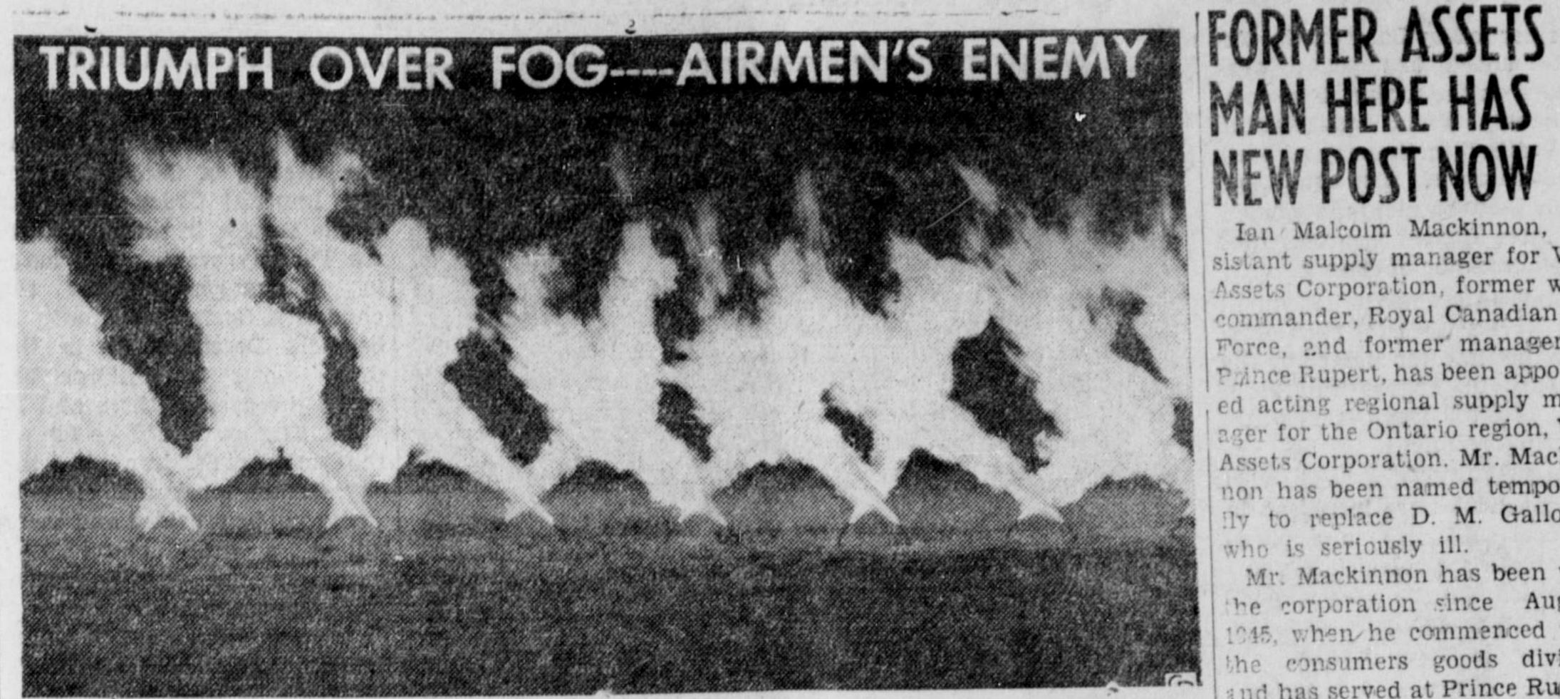
FOG-FIGHTING FIRE-Tongues of flame, seven feet long, blaze against the night sky as a series of diesel oil-burning fog dispensers hurl their barrage of super-heat into the air to
