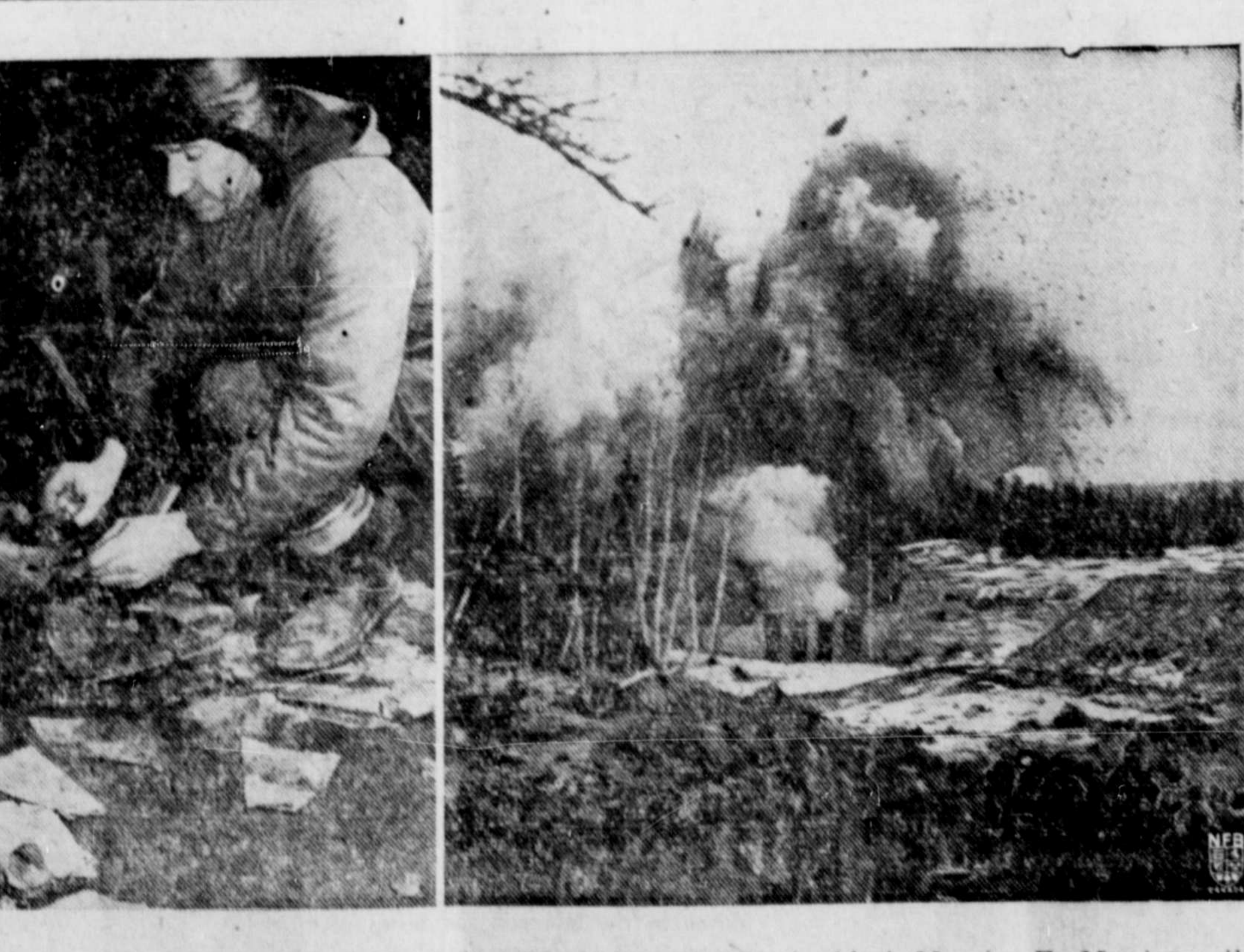
BLAST REVEALS ORE BEDS—To reach the rich iron ore beds at the bottom of Steep Rock Lake in northwestern Ontario, more than 121,000,000 gallons of water had to go "down the drain." So this could be done, 15 tons of dynamite were used to divert water from Marmion Lake, which fed Steep Rock. The first picture (left) shows Arthur Dymont and Frank Jones of the C. A. Pitt Construction Company, examining the wiring prior to the blast. Maurice F. Massiaen, the firm's mechanical superintendent, touched off the blast (right) sending heavy logs flying more than a mile and great chunks of rock high into the air. After the 608 cases of dynamite blew, the Marmion Lake outlet was running west instead of southeast.
