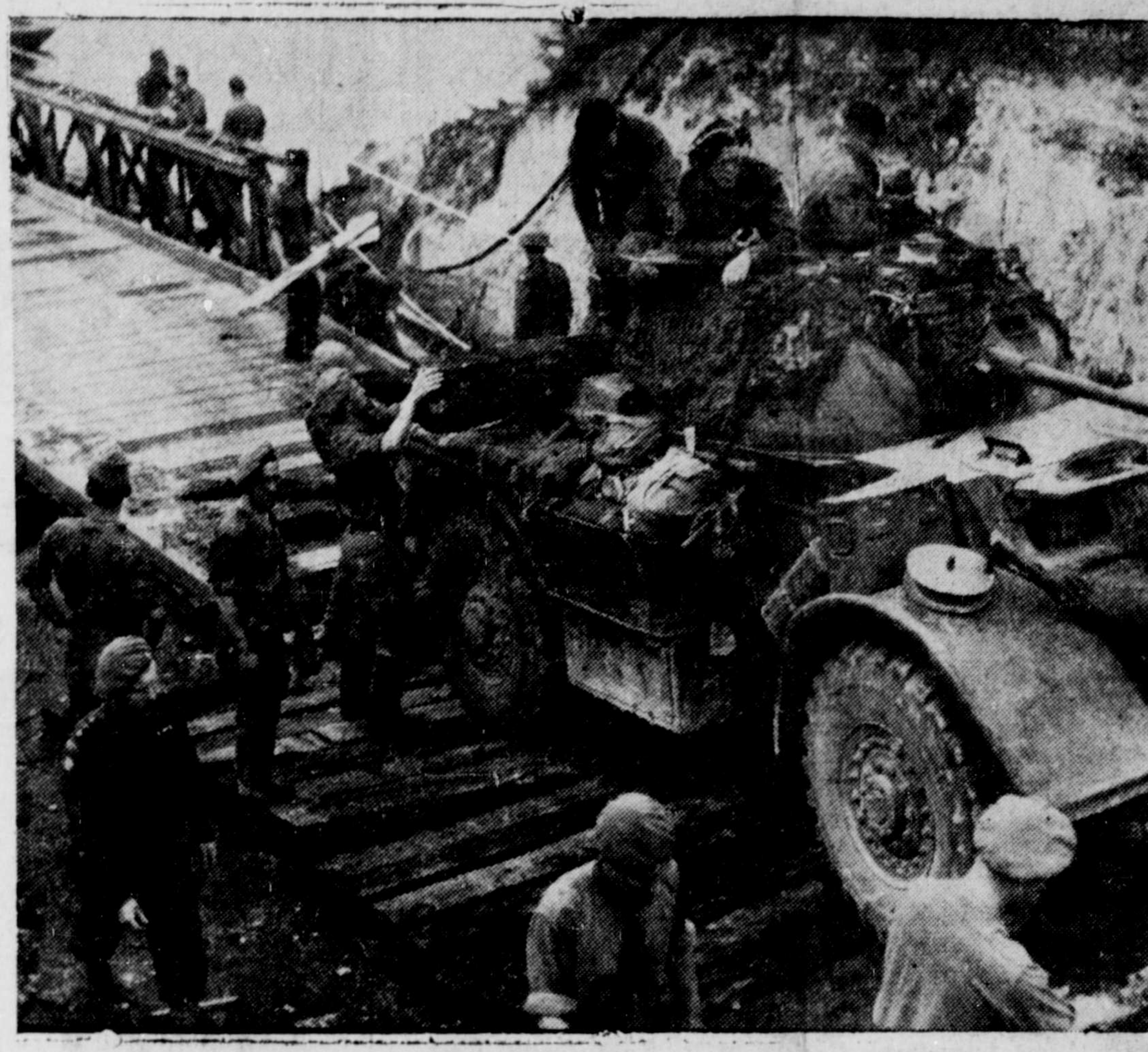
CANADIANS CROSSING THE SEINE—Over a hastily constructed Bailey Bridge these Canadian vehicles loaded with railway ties, cross over the Seine. The ties were used to reinforce a fresh clay roadway in record time by the Royal Canadian Engineers.
