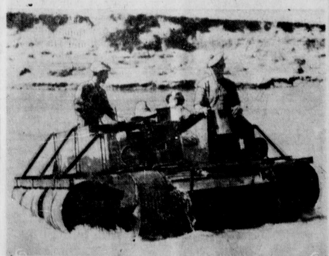
BRITISH ENGINEERS of the 14th Army devised this ingenious method of getting a Bren gun carrier across the Mu river during the drive on Mandalay. Large oil and gasoline drums were strapped to the vehicle to keep it afloat. Motive power was supplied by the carrier's caterpillar tracks acting as paddles.
