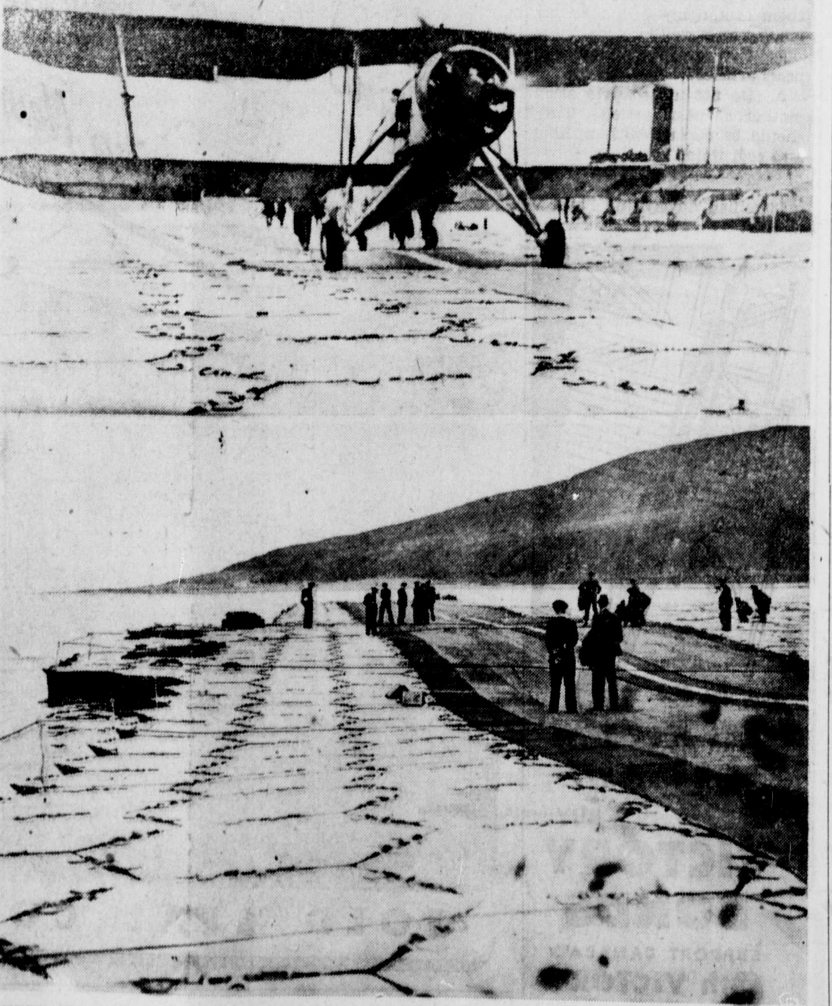
HERE IS THE "LILY," BRITISH PORTABLE SEADROME — Just released from the British secret list is the "Lily," portable seadrome invented by R. M. Hamilton, who was a Royal Navy petty officer at the start of the war. It consists of a number of buoyancy cans with hexagonal surfaces, so linked together that they can give in a controlled manner, to the motion of the sea from any direction, and yet remain sufficiently rigid to take the weight of heavy aircraft. A Swordfish (above) lands on the "Lily" leaving a depression on the surface. The "Lily" undulates with the waves (lower photo) as a motor launch passes at high speed.
