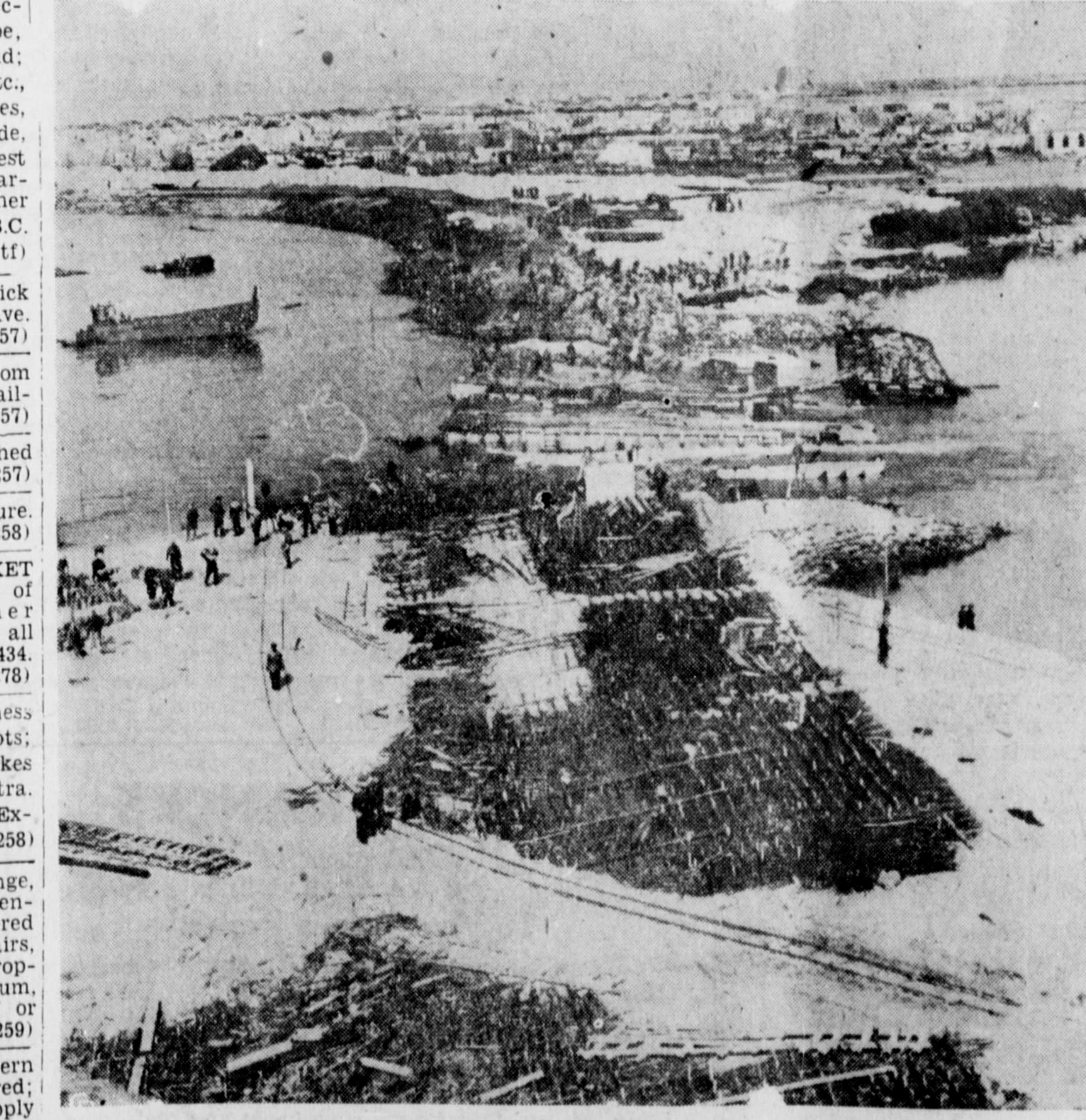
WALCHEREN RISES FROM THE SEA AGAIN—Literally "sunk" when its dykes were breached by the Nazis during the invasion by the British about a year ago, Walcheren Island, off the Holland coast, is being reclaimed from the sea by Dutch workers with British aid and equipment. A breach in the sea-wall is here being closed by sinking specially-built barges and adding a rock fill. After the inlets from the sea are closed the great task of pumping out the water will begin.
