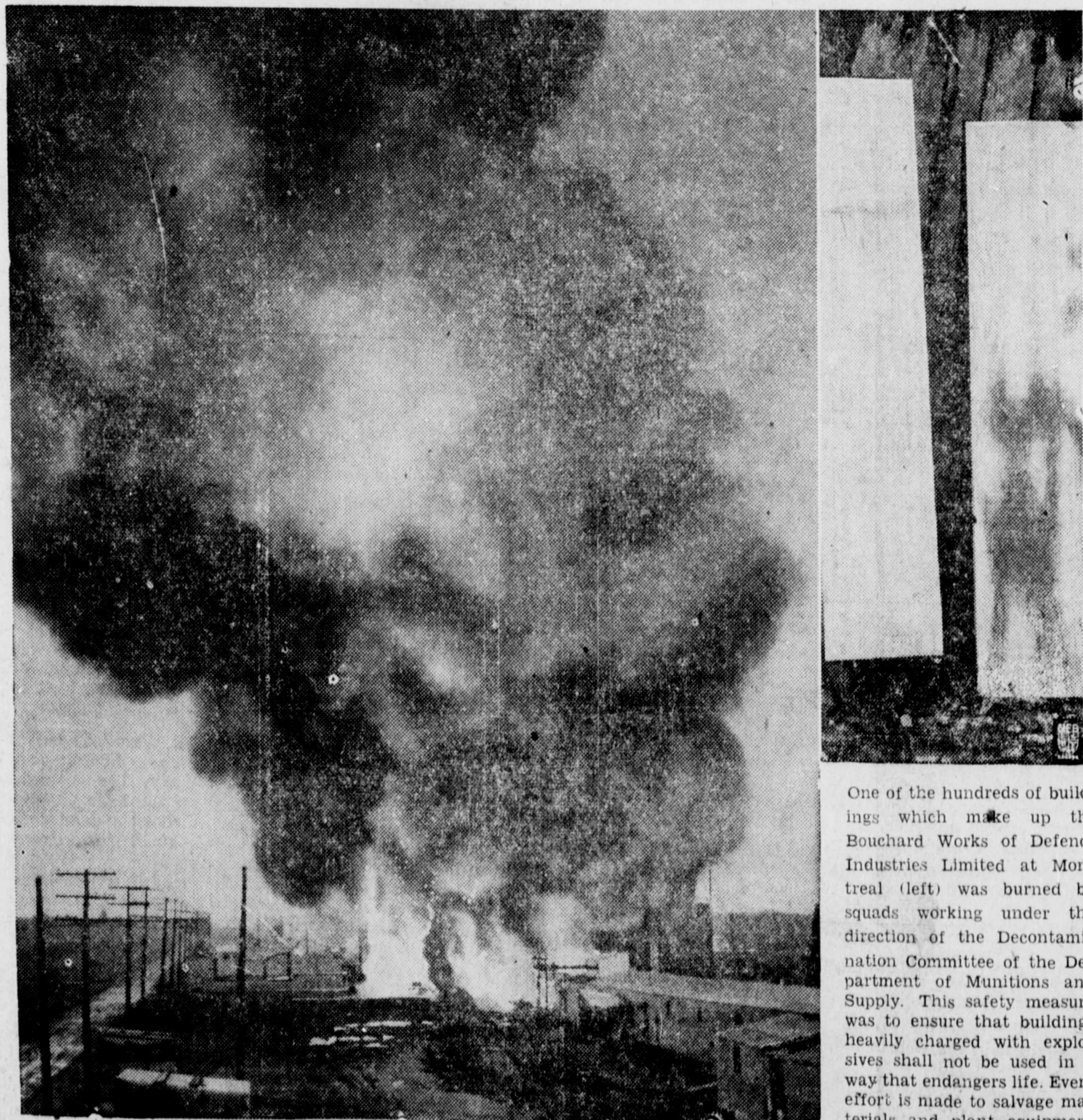
Corporation. Pieces of wood from structures at Defence Industries Limited (right) show one of the tests to detect the presence of explosives. Chemical compounds are poured or sprayed on the material; if the wood does not change color, the explosives are not present, but if it turns pink or red, explosives are imbedded in the fibres of the wood and are combustible.
