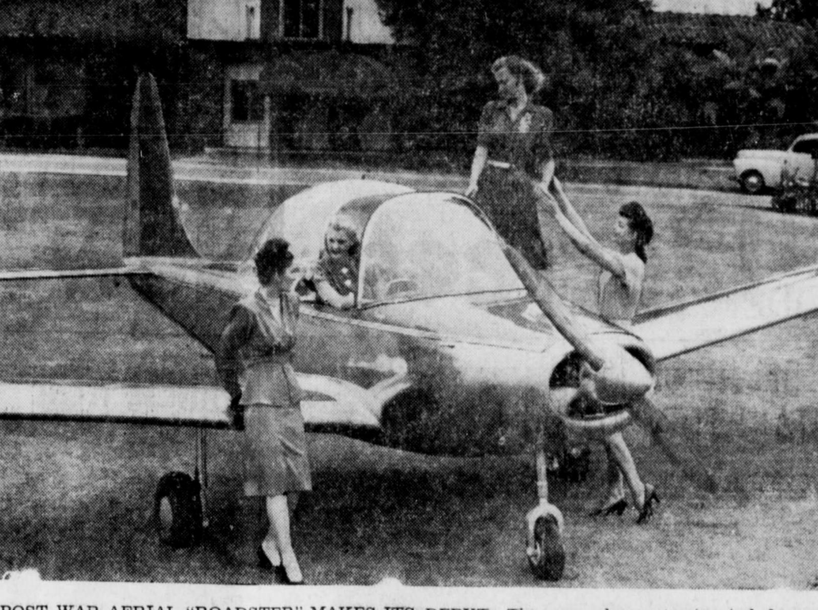
POST-WAR AERIAL "ROADSTER" MAKES ITS DEBUT-The new plane, constructed for private use by American Aircraft Inc. is called the "Ensign" and is a two-place low wing mono-Always fresh-at your grocer's plane of all-metal construction within the price range of a high-priced automobile (\$3,000). It has seat and dashboard designed like an auto and full vision enclosure. Four-some of girls give the Ensign plane the onceover. Left to right are Norma Krieger, Toni Barron, Ruth Allen and Sheryl Mitchel.
