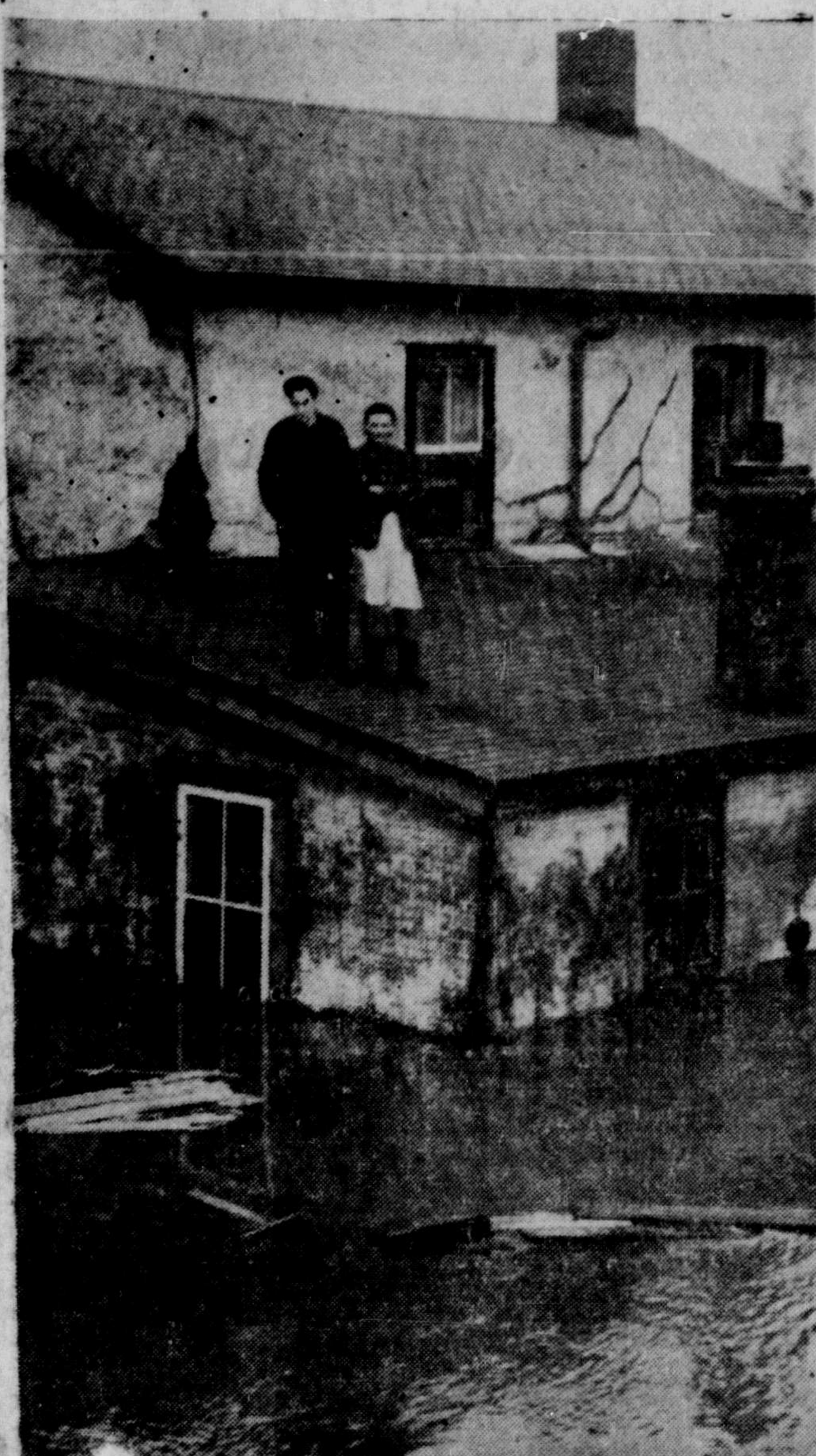
ONTARIO RAVAGED BY FLOODS, Brampton, Ont., was missed by the Etobicoke Creek when it went on the rampage, wrecking the entire business section. Mr. and Mrs. Bert Forrest were forced to climb on the roof of their home to await rescue.
