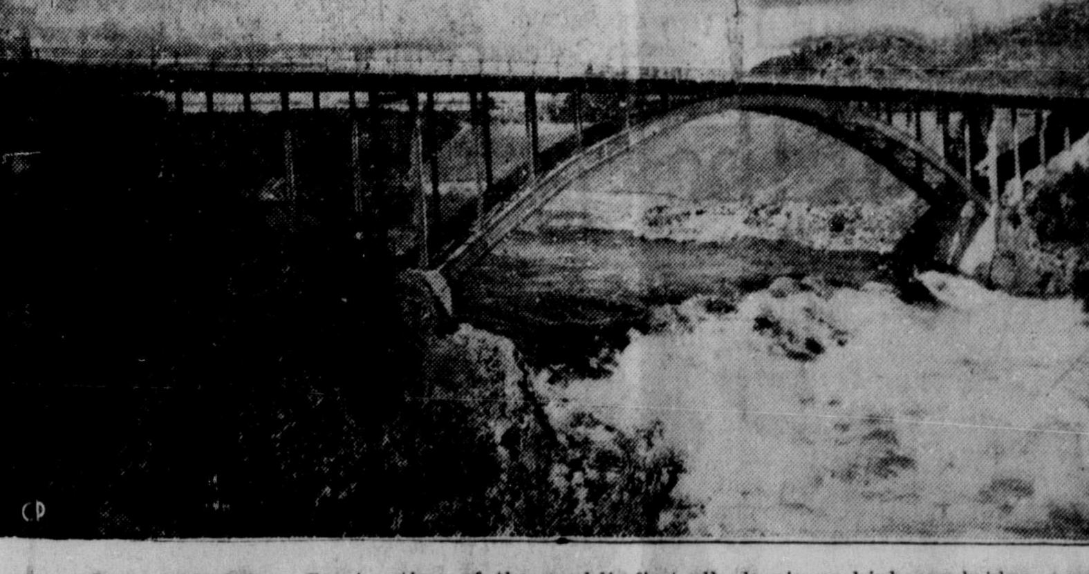
ALUMINUM BRIDGE - Construction of the world's first all-aluminum highway bridge, across the Saguenay River between Arvida and Ship haw in northeast Quebec, has been completed. The \$500,000 structure is close to Canada's big aluminum smelter at Arvida. An aluminum bridge was opened in Sunderland, Eng., last year, but unlike the 504-foot Arvida structure, it is a railway bridge.
