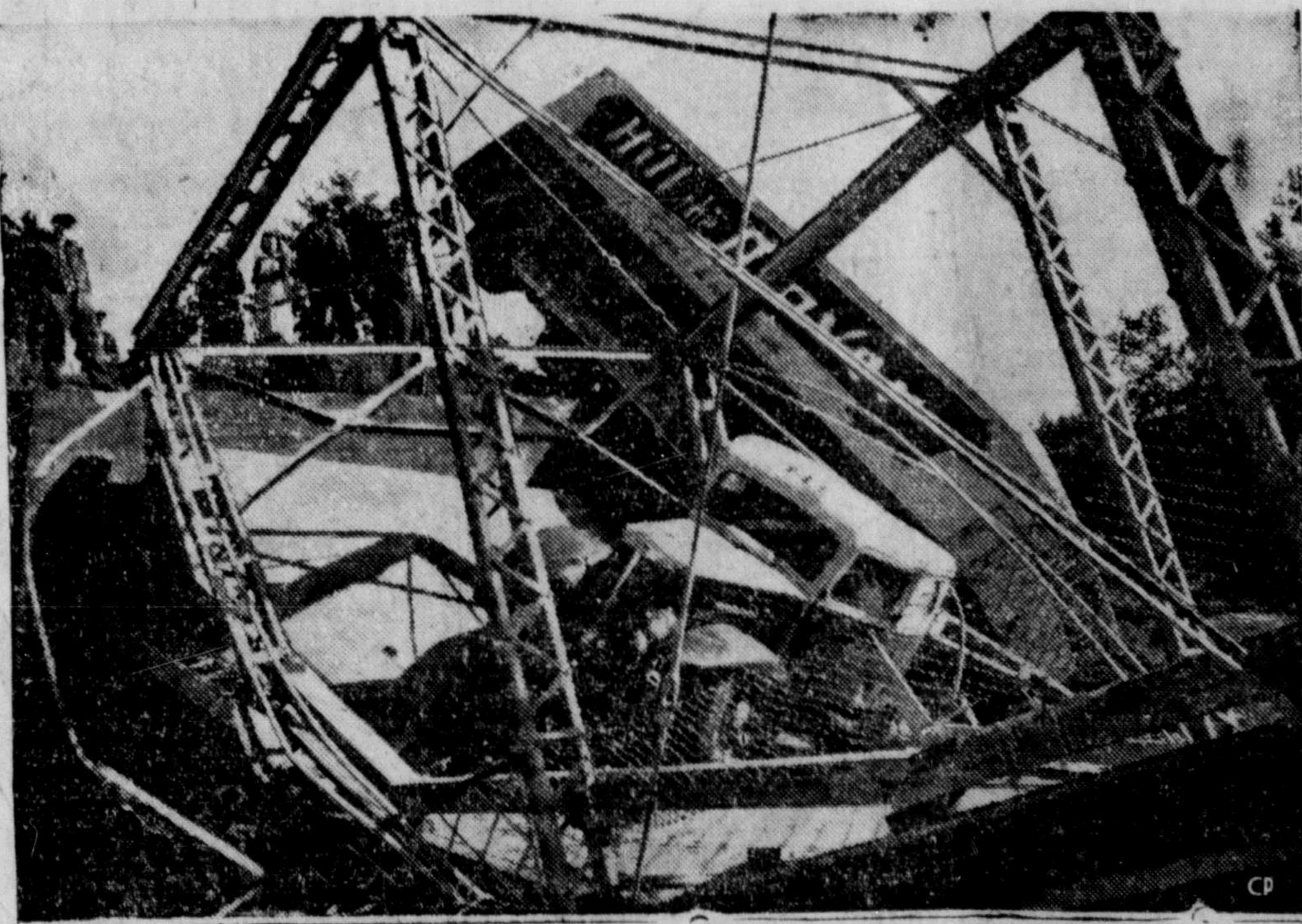
LUCKY ESCAPE—Two Toronto men, riding in this truck, escaped serious injury when the big transport dropped through the Maclean River bridge near Southampton, N.S. Even the truck was little damaged. It is believed the bridge slipped off its cribs just as the vehicle started to cross. The bridge was a complete loss. (C. P. Photo)
