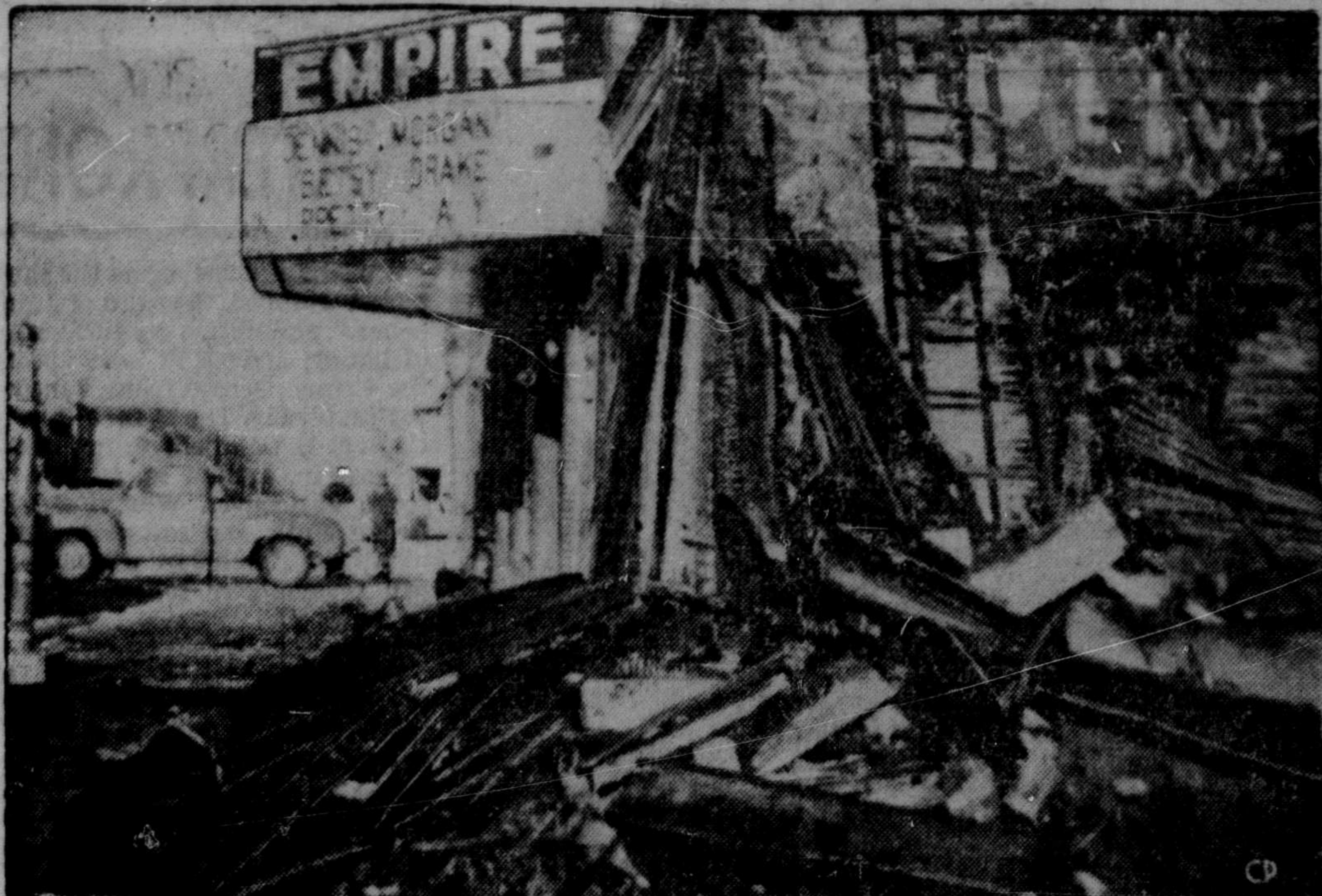
WALL SAVES THEATRE —Only a thick brick wall saved the Empire Theatre as flames engulfed four adjoining business blocks in a $500,000 fire in Thessalon, Ont. No one was injured, but 15 persons were made homeless. (CP PHOTO)
