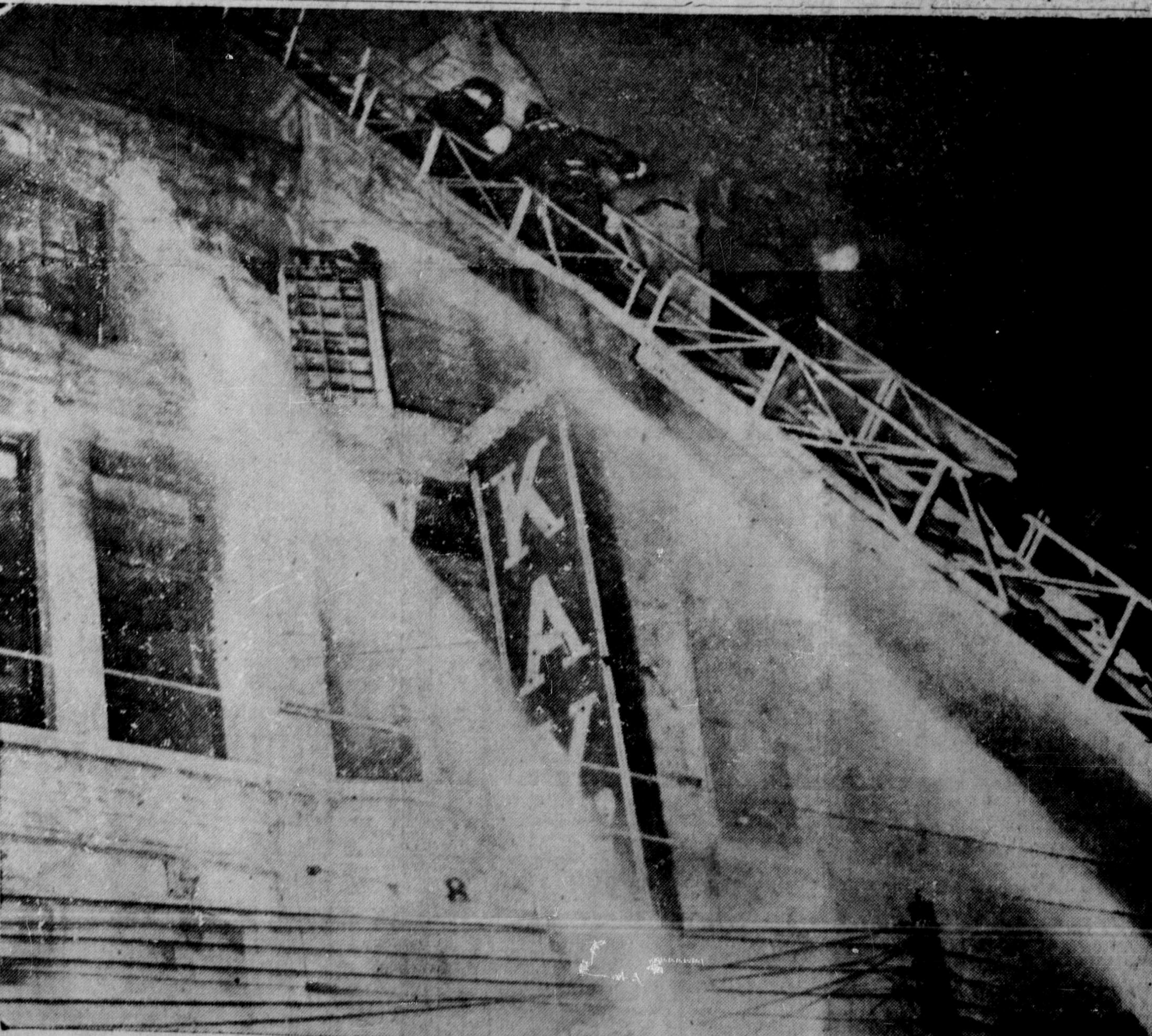
WHERE 10 DIED —A toyland fire in Kay's department store in downtown Halifax, which broke out shortly before closing time, claimed the lives of 10 shoppers and clerks late Thursday afternoon. Fire spreading from a display window cut off the
