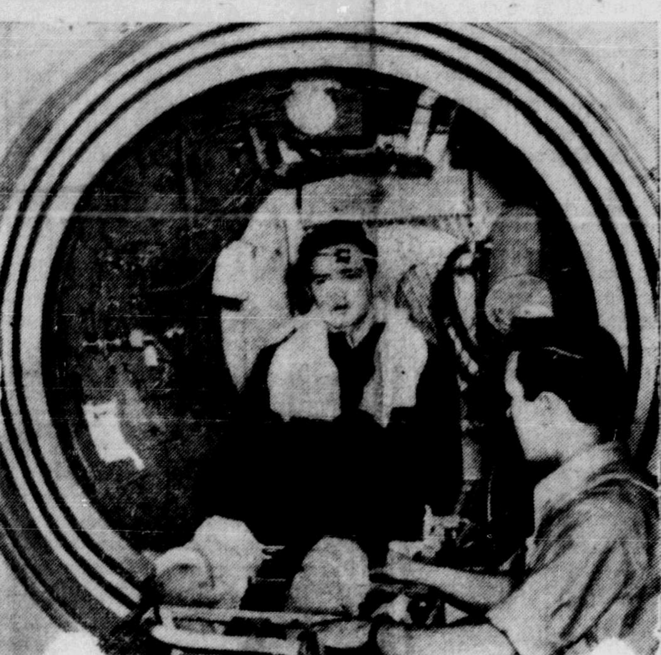
BOILED FOR THE SAKE OF SCIENCE —Using themselves as guinea pigs, six scientists at the University of California at Los Angeles have cooped themselves up in a sealed room considerably hotter than boiling water, to prove that pilots would be able to stand the intense heat generated by friction when airplanes hit 1,000 miles per hour. They proved that the human body can stand temperatures up to 250 degrees Fahrenheit, which is 38 degrees above the boiling point of water. For periods of fourteen and a half minutes the scientists, headed by Dr. Craig Taylor, took turns in the chamber. One of the student volunteers, Si Friedlander, is pictured being removed from the heat chamber after he was subjected to the test.
