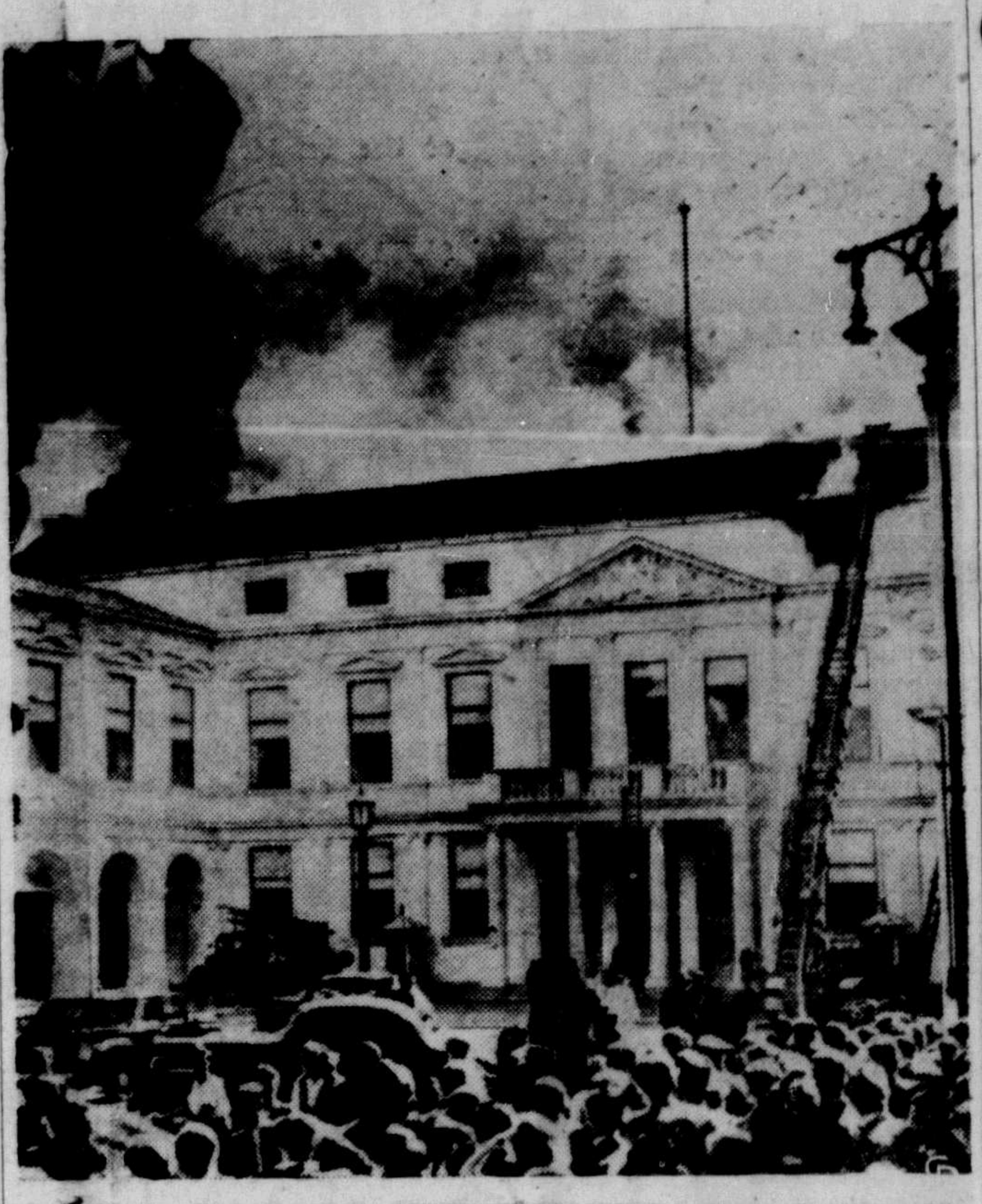
QUEEN'S APARTMENT GUTTED BY FIRE—The private apartments of Queen Wilhelmina of Holland were gutted by fire in her Noordeinde palace at Houe. She was not in the residence at the time but Prince Bernard, husband of Juliana was there and directed the removal of treasures while fire fighters fought the blaze.
