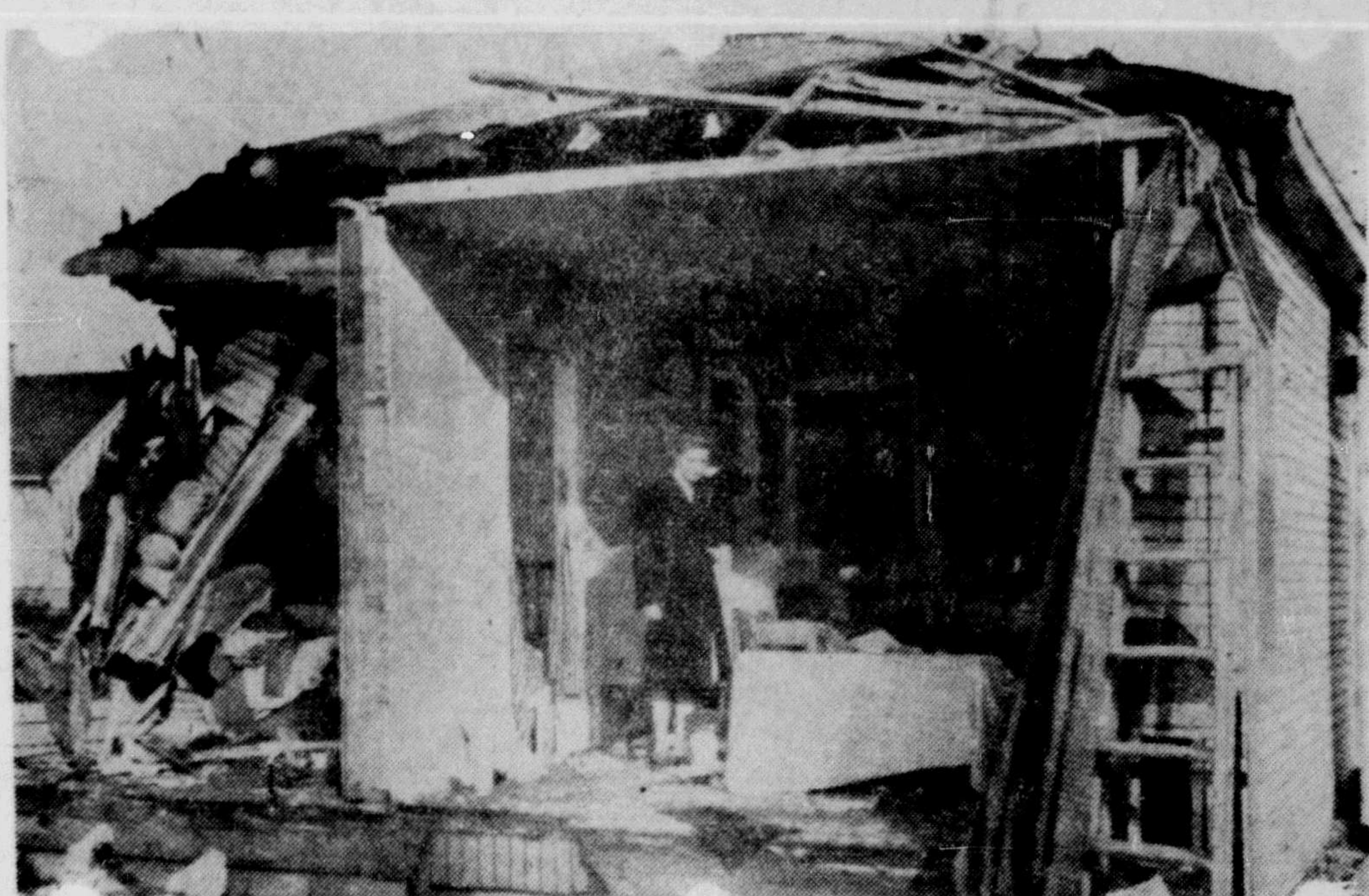
TORNADO CAUSES WIDESPREAD DAMAGE IN MIDWESTERN STATES — An unidentified woman (above) is shown standing amidst the ruins of her home at Porter, Indiana, after it was ripped apart by the tornado which swept through sections of Illinois, Indiana and Kentucky. Five persons were reported killed and many injured by the twister, which inflicted heavy property damage.
