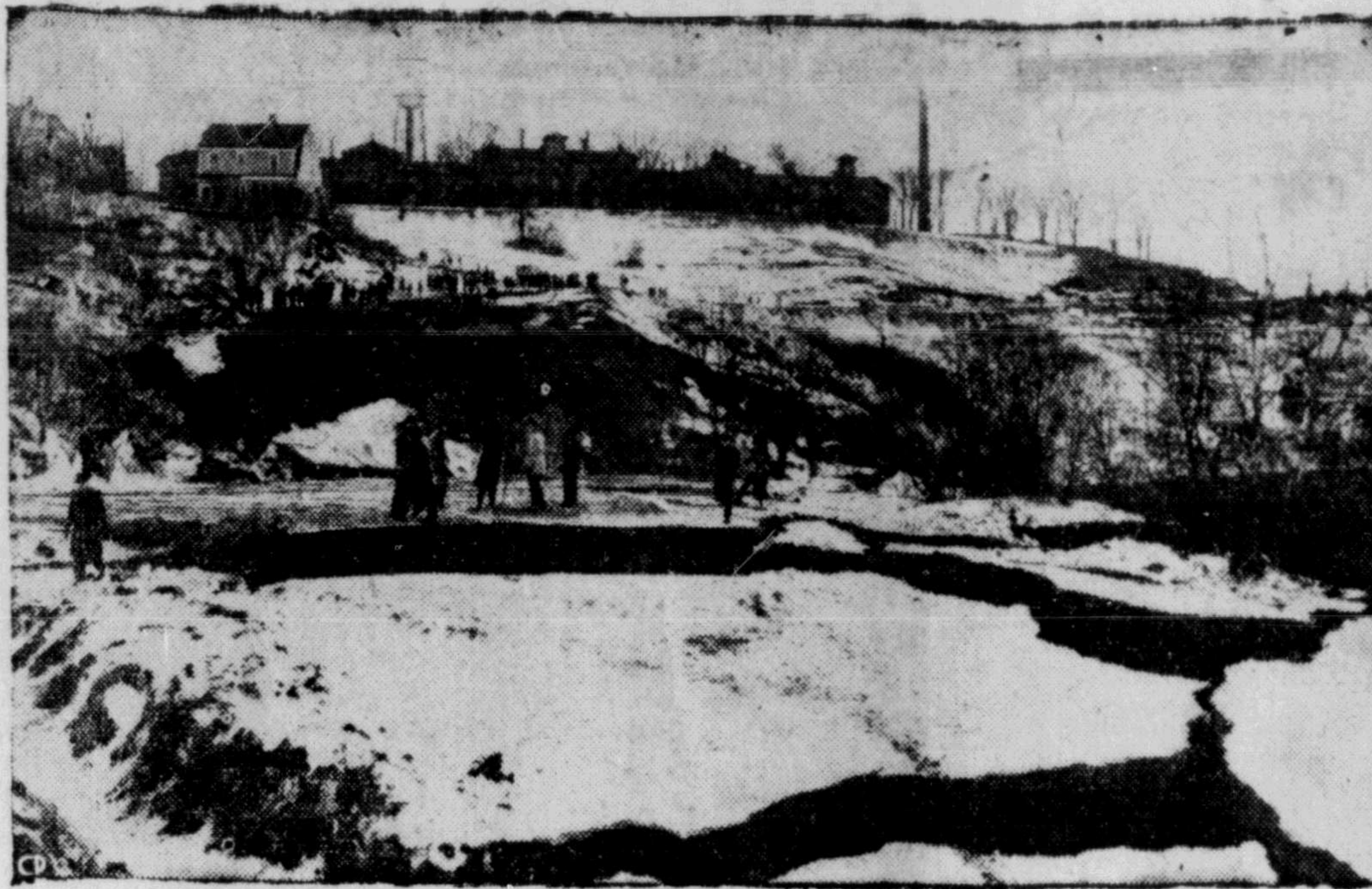
ROAD DISAPPEARS —Land settling on Lancaster Avenue in Saint John, N.B., is creating these gaping fissures in what used to be a scenic drive bordering the city's famous reversing falls (far right). One section of the road (foreground) is 60 feet below its original level. In the left background is part of a 90-foot high cliff carved when thousands of tons of earth dropped toward the harbor basin. On the second "island" engineers measure the sinkage. (CP Photo)
