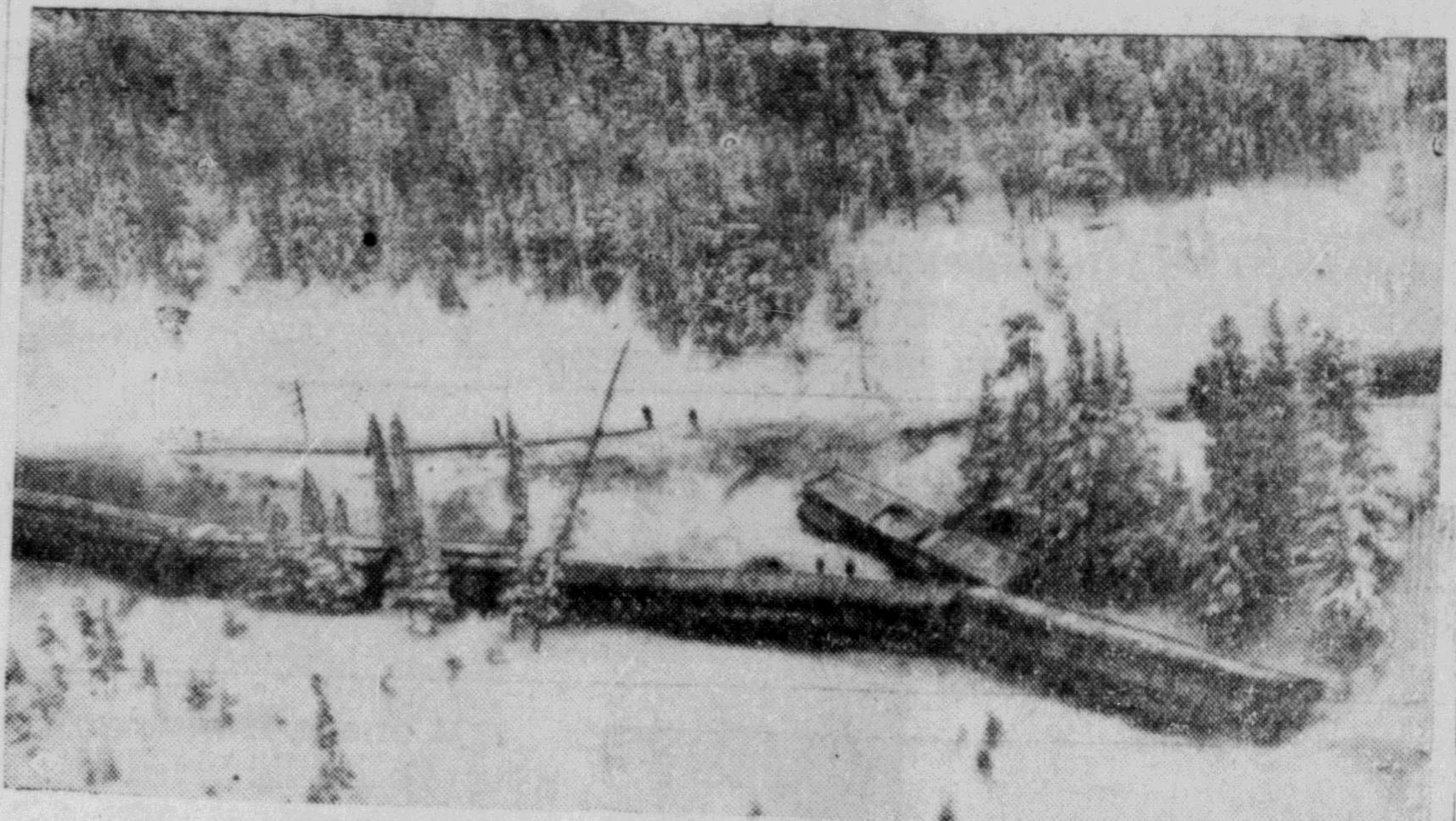
CRACK TRAIN DERAILED —A broken rail is believed responsible for the derailing of the C.P.R.'s crack Dominion three miles east of Banff, on January 18. One person was seriously injured and more than a dozen others suffered minor injuries. This aerial photo shows the cars strewn along the main line after leaving the rails near a sharp curve. (CP Photo)
