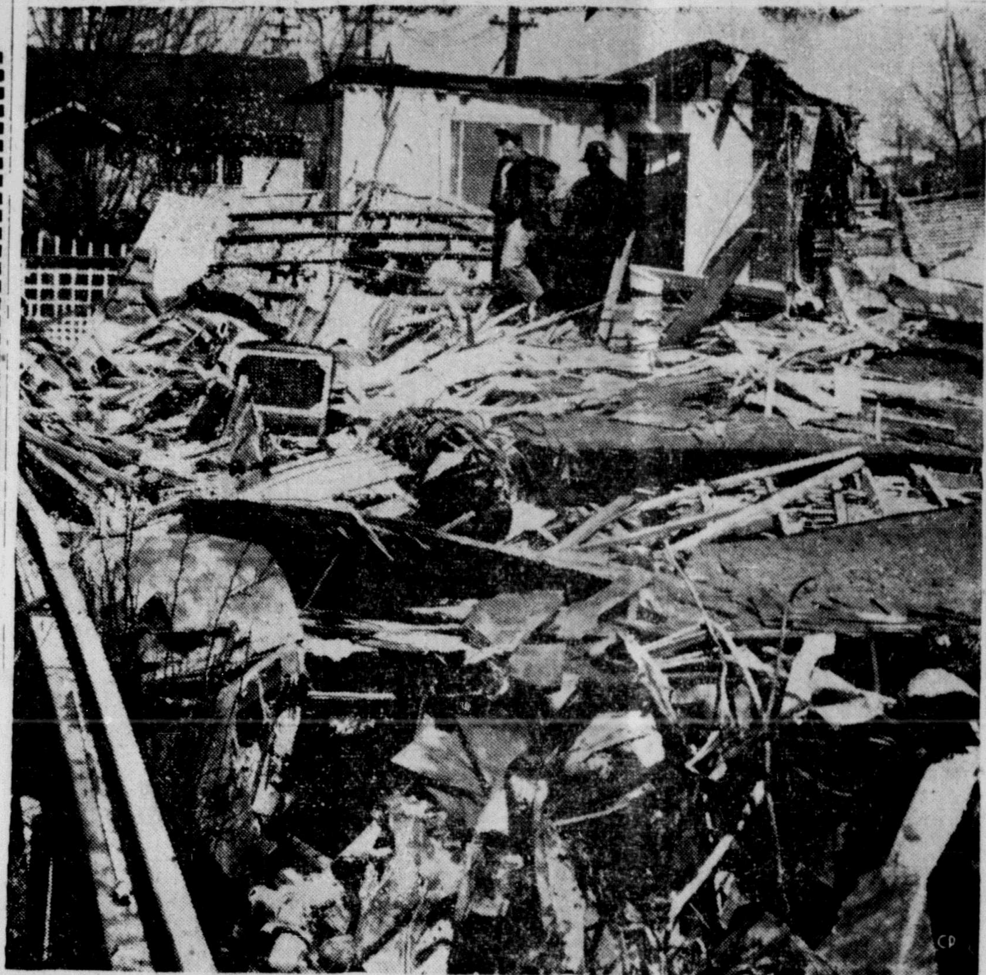
NARROW ESCAPE —The four occupants of this house escaped severe injury when the five-room bungalow on Calgary's North Hill was demolished in a plane crash. Jack Harper, 22-year-old pilot of the twin-engine Cessna, was instantly killed. Police said they were told by witnesses that Harper, a salesman for an aviation company, had been drinking before he took one of his company's planes on the night-time rooftop-hopping flight. Shown in the background centre is the last remaining wall of the house of Marshall McDougall, a police station switchboard operator. The debris in the foreground includes both the plane and the house. (CP Photo)
