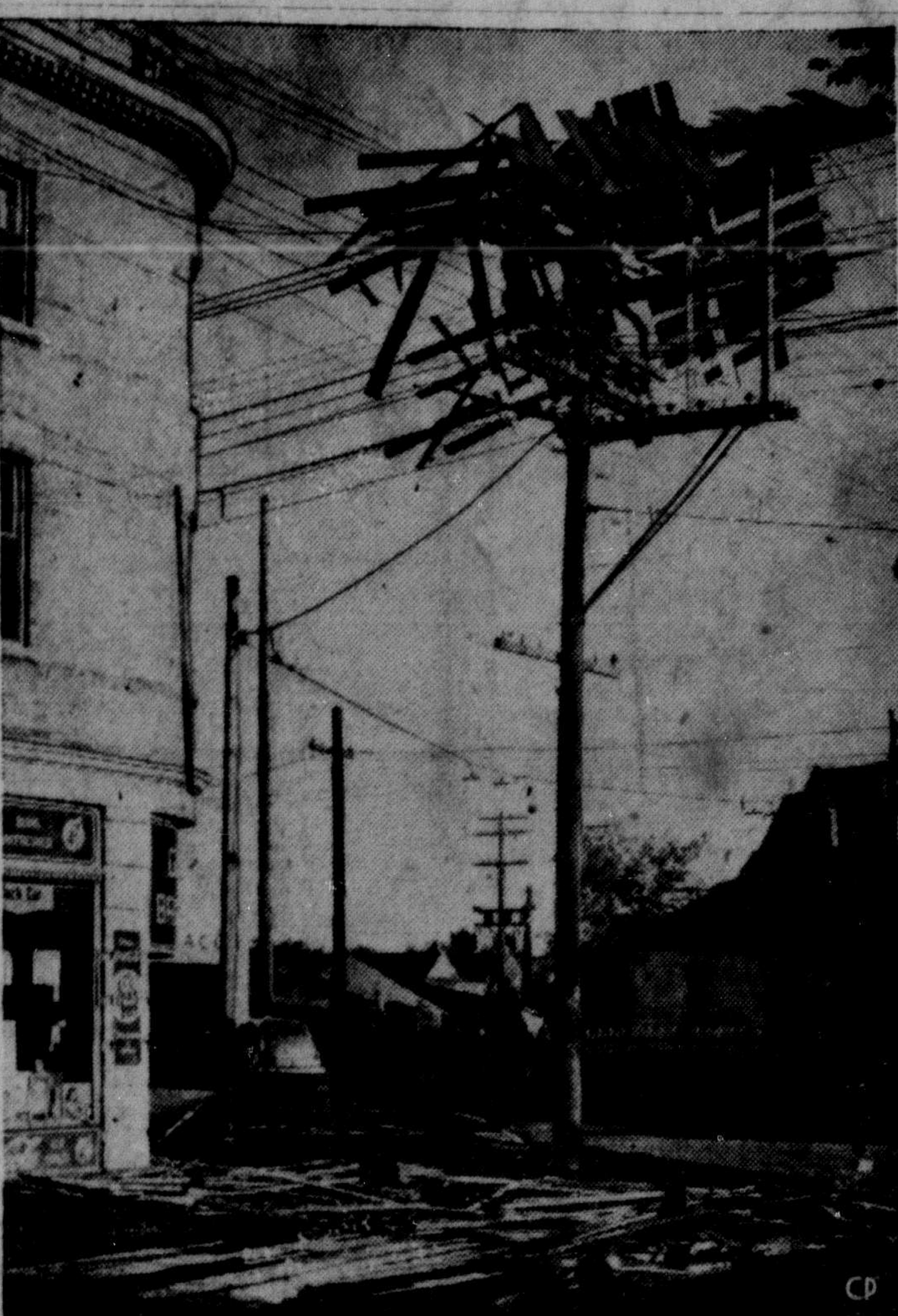
STORM AFTERMATH—Not a shelter from the wind for telephone line workers, but the roof of an apartment house deposited here by a wind of near-cyclone force which swept Winnipeg Monday. The wind accompanied by heavy rain caused considerable damage to the Manitoba capital still recovering from the disastrous Red River floods of May. (CP Photo)
