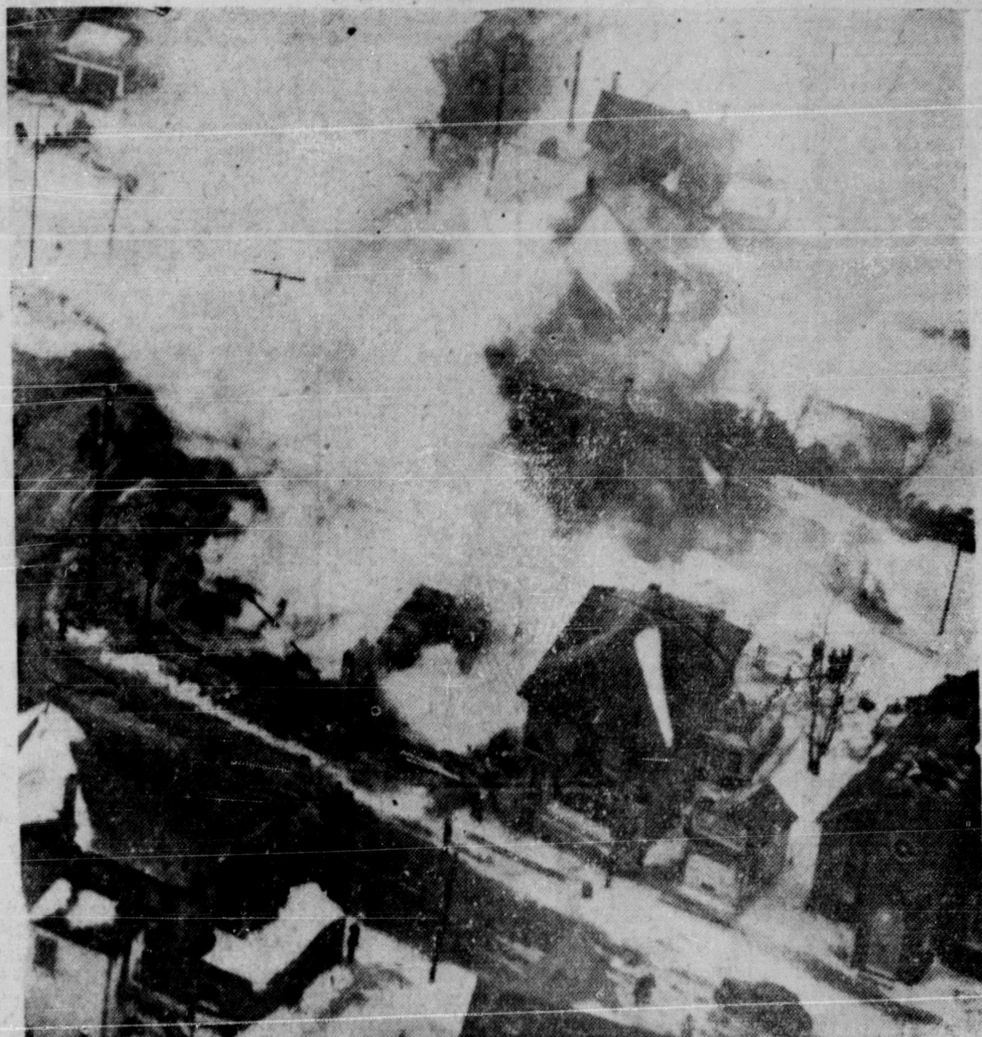
$130,000 FIRE—Fire which raged for three hours through the business section of Sunderland, Ont., caused damage estimated at $130,000 last Thursday morning.
