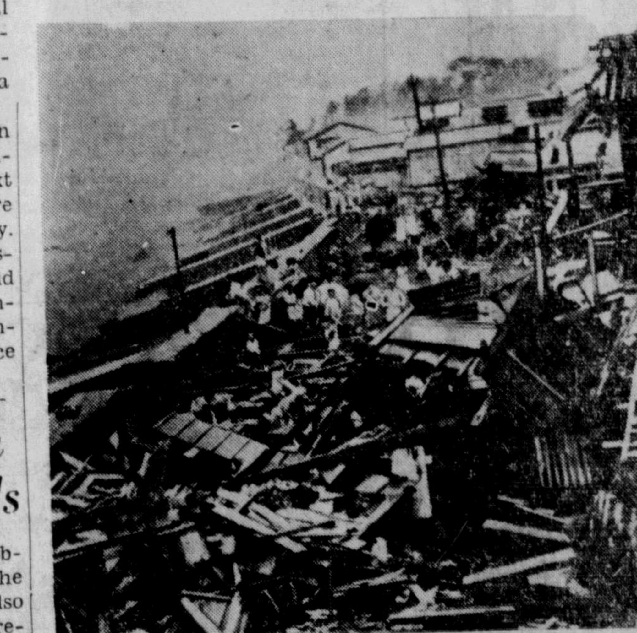
AFTER THE TYPHOON STRUCK—Wreckage of homes and buildings strewn along the banks of the Tone river marks the path of the disastrous typhoon "Kitty" that swept Japan's mainland island of Honshu last week. The big wind and resultant floods left 144 persons dead or missing, thousands homeless and damage to property running into the millions.
