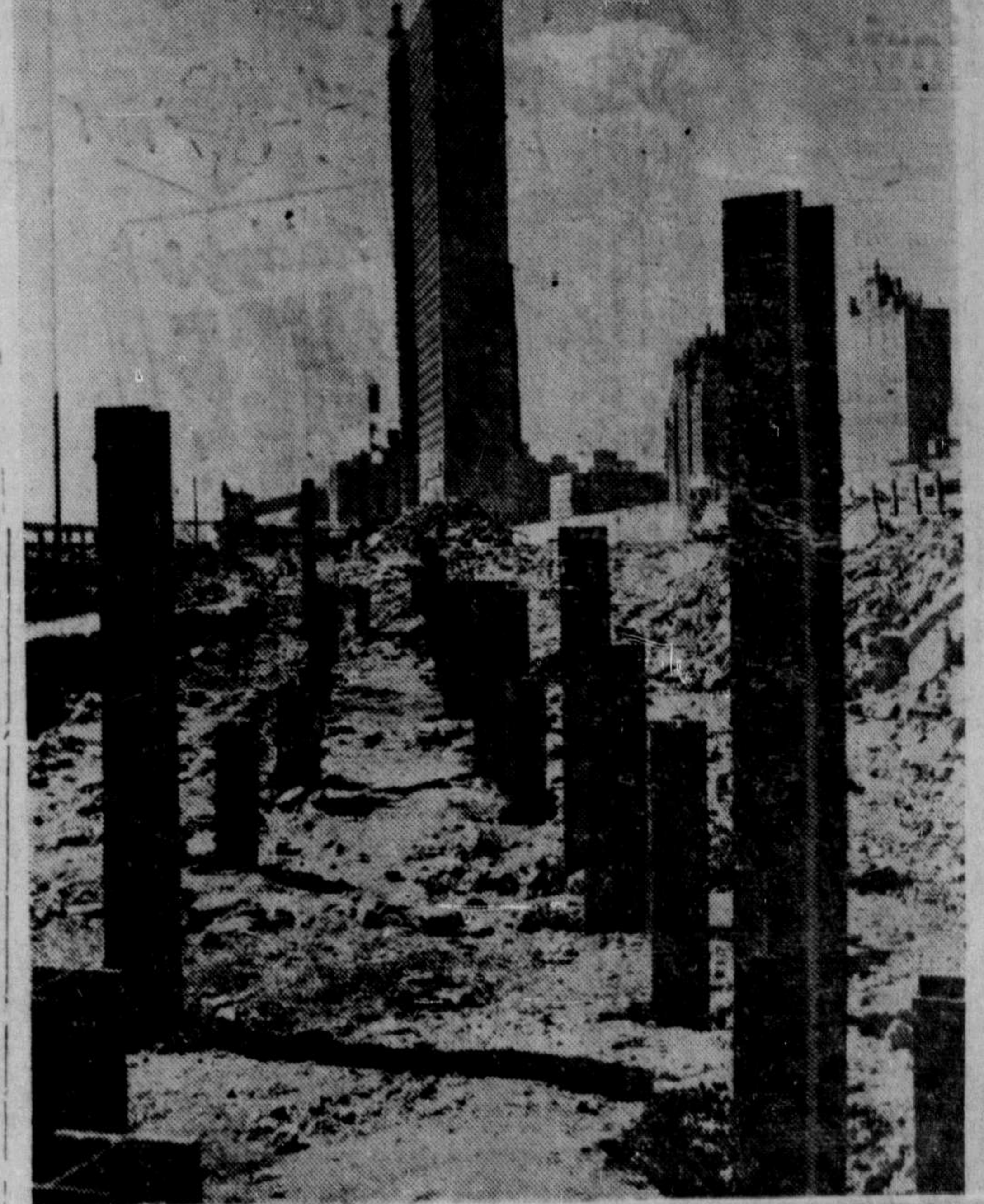
U.N. BUILDING ALMOST READY FOR USE—This striking view of New York's United Nations secretariat building, which is practically ready for occupancy, shows the towering skyscraper moment to peace, through rows of steel posts which could be taken for graveyard markers. The posts are being driven into the ground for new buildings and a roadway that will form the approach to the building.
