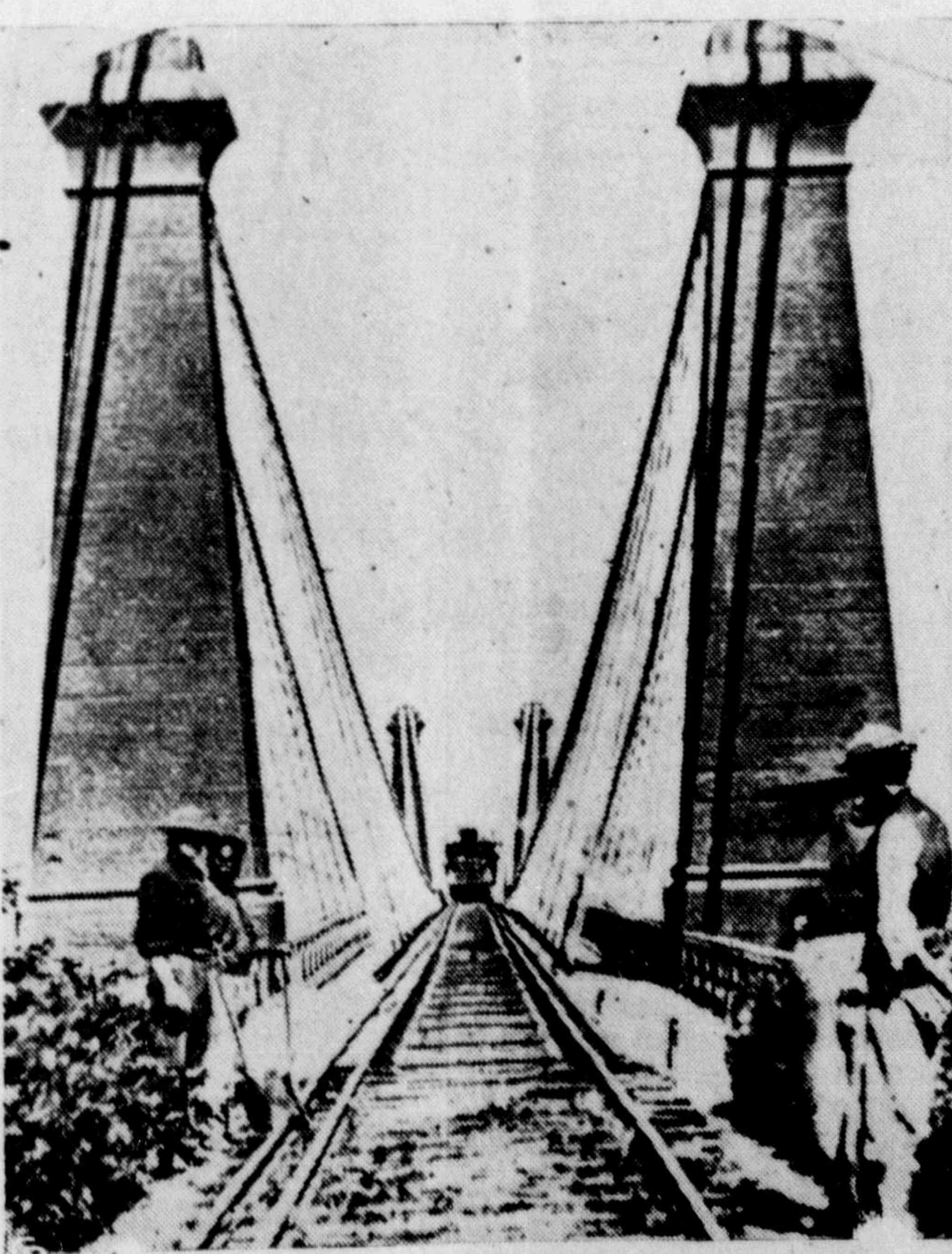
WHIRLPOOL CENTENNIAL BRINGS BACK MEMORIES—The Whirlpool Rapids Bridge Centennial at Niagara Falls this week revived a century of memories. In the 1870's it took three rails to get trains across the bridge. Note third rail inside the two standard tracks to accommodate old narrow gauge wood-burners, in this picture of pioneer Whirlpool Rapids Bridge.
