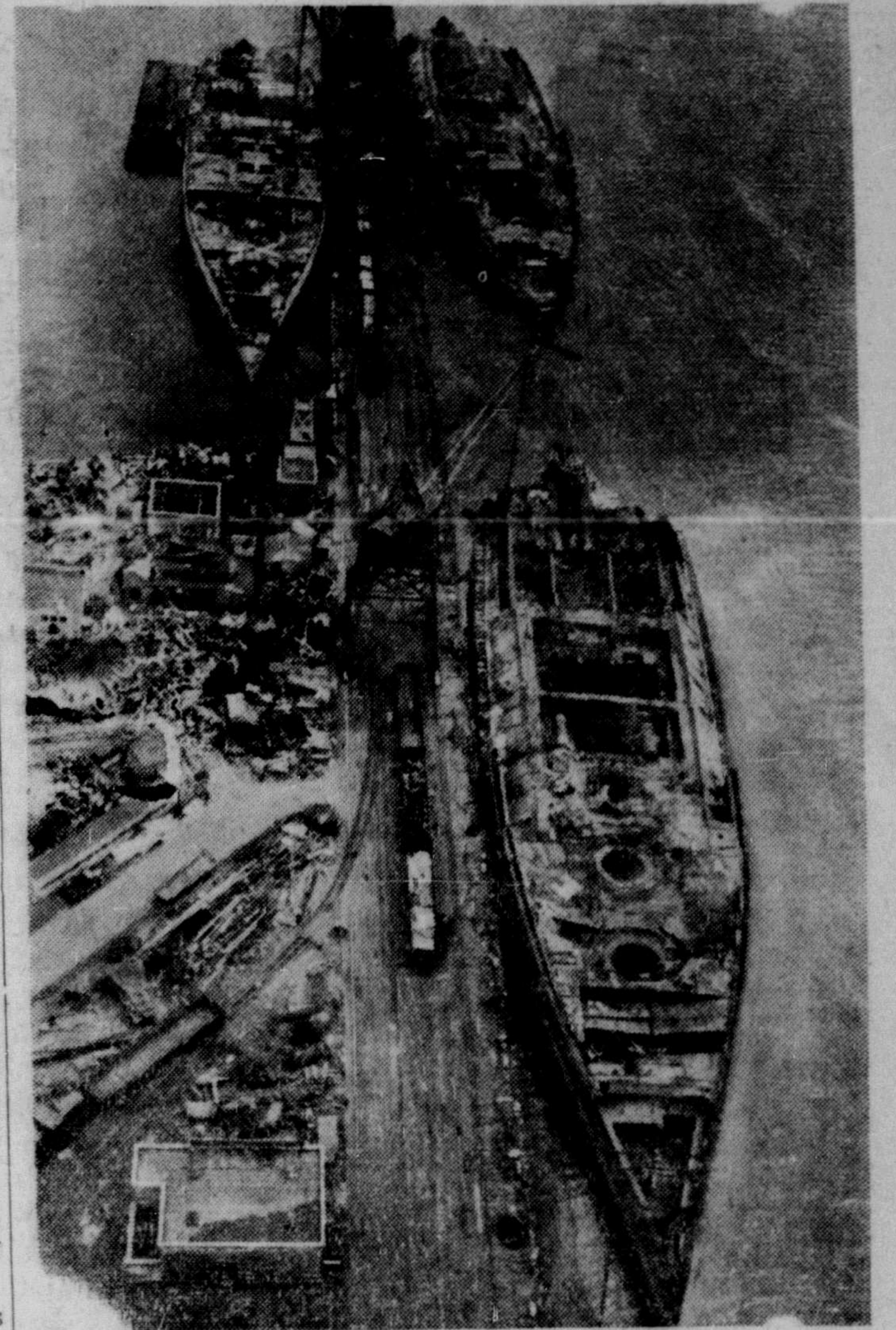
FROM SEA VICTORIES TO SCRAP METAL—Fast being reduced to scrap metal, three mighty U.S. warships are shown in this air view as they were being stripped at Pt. Newark, N.J. At upper left is the Wyoming; upper right, the Idaho and, lower right, the New Mexico. The Wyoming was expected to supply 15,000 tons of scrap and the three ships were expected to yield 57,000 tons.
