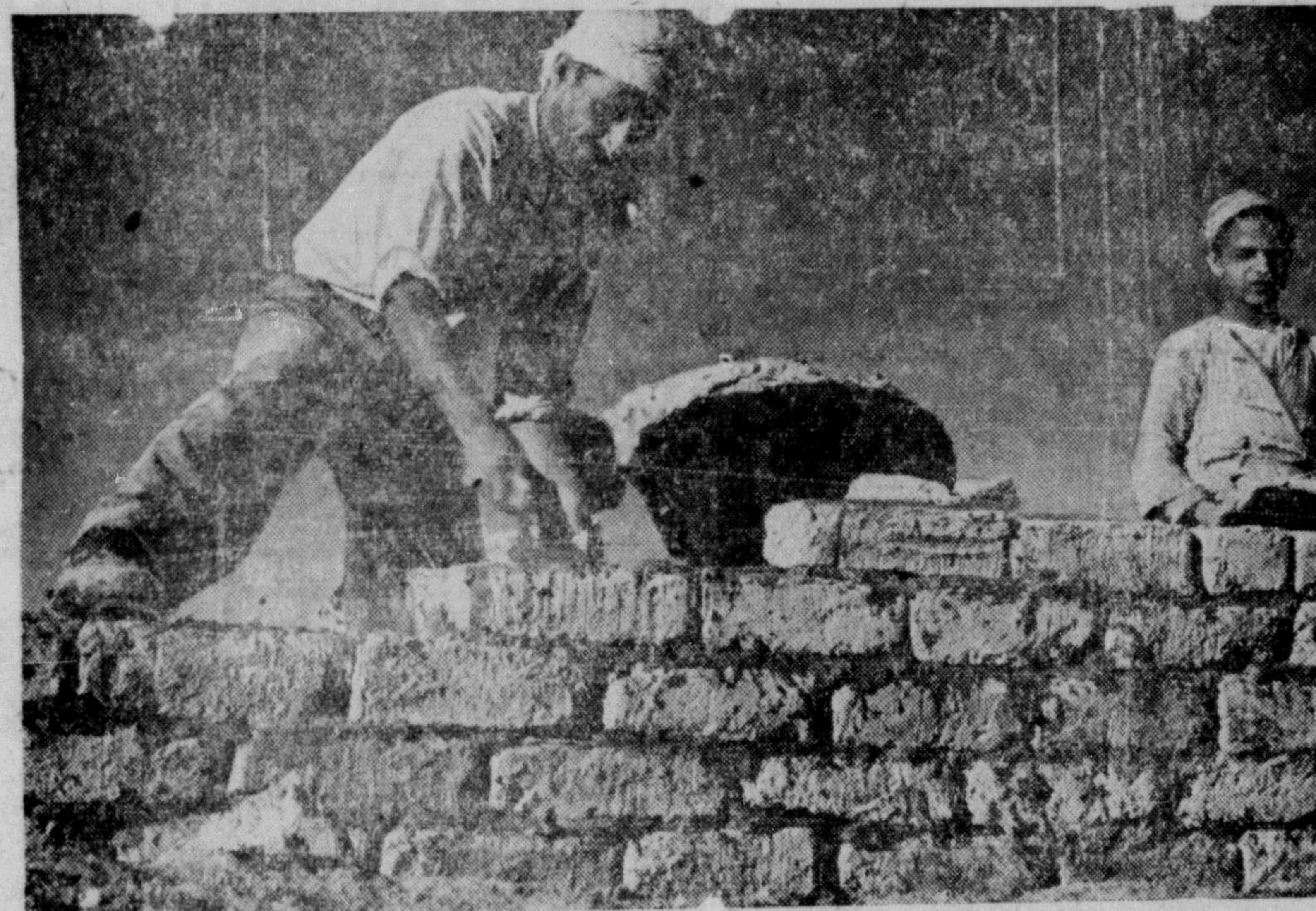
ON THE CREDIT SIDE OF THE UNITED NATIONS' EFFORT —United Nations' conferences seem to be getting nowhere, but in many places throughout the world, the U.N. effort is bearing fruit. Here an Arab refugee, made homeless by the Israel war, builds his home of mud bricks with the aid of his son. United Nations funds and experts are helping to make whole new villages for the refugee Arabs.
