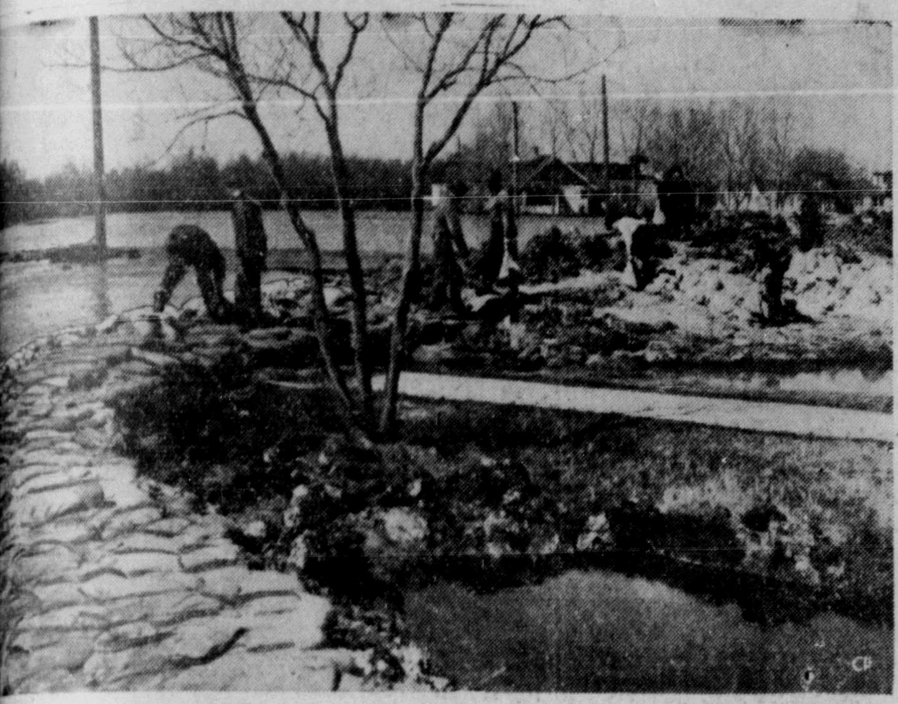
FLOOD SPOT —Rough winds buffeting flood water against a line of sandbags at the Fort Garry dike crossing the Pennington Highway in Greater Winnipeg have been termed "extremely noisy" by army engineers. Feverish activity to build up the dike can be seen as men pile bag after bag against the wall of water. (C P Photo)
