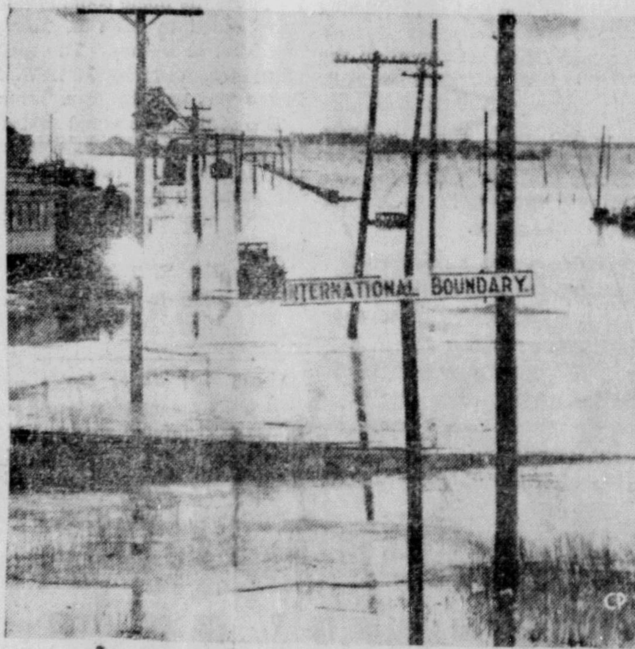
WATER CURTAIN —Europe has its Iron Curtain. Just now there's a watery counterpart between Canada and the United States in southern Manitoba. This is the International Boundary at flooded Emerson, Man. Motor traffic is impossible but trains are getting through. (CP Photo)
