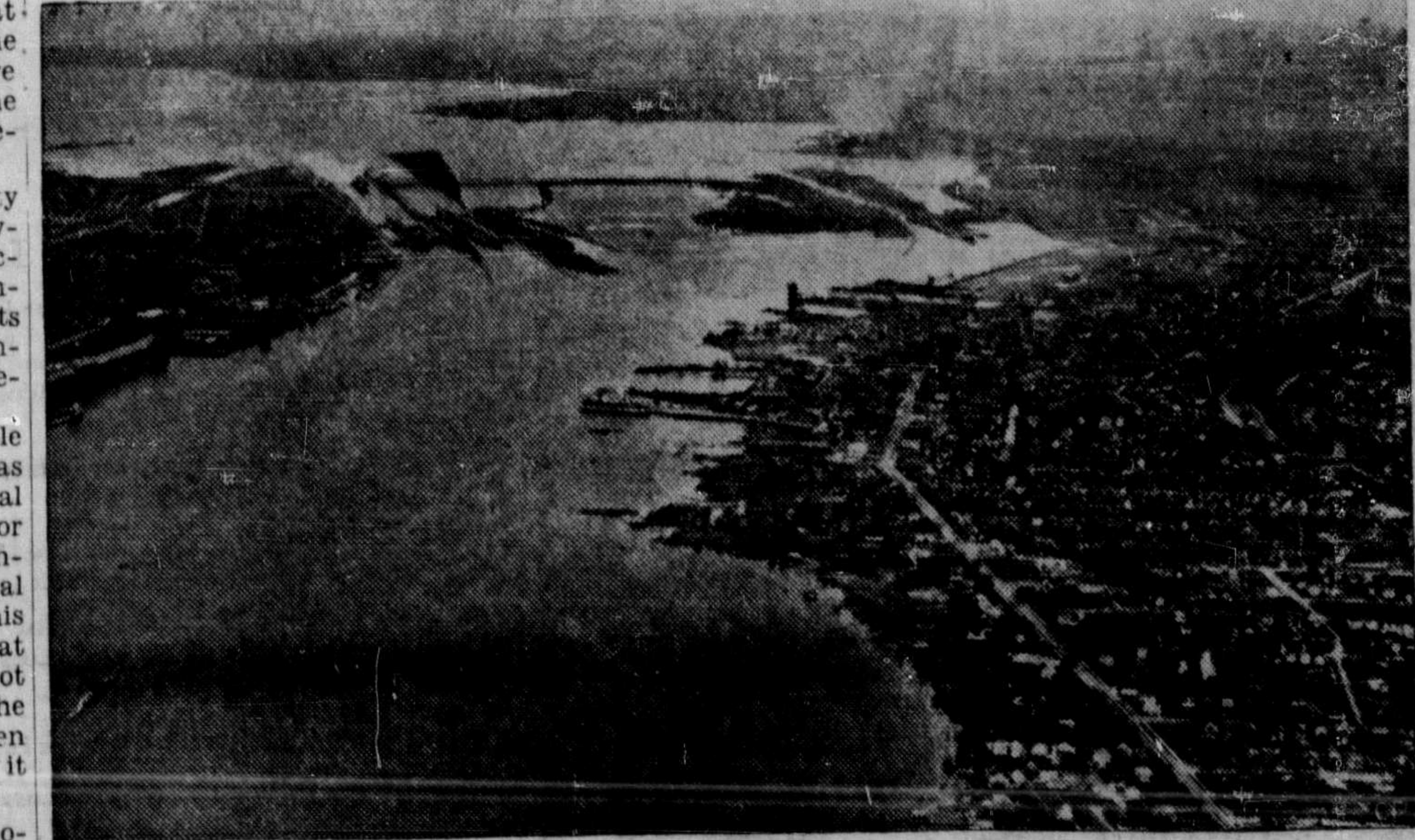
THIS IS AN AERIAL VIEW of the world's busiest canal system, which bypasses the rapids of the St. Mary's river and which in 1953 cracked its own cargo record. Four canals are on the United States side of the river and one on the Canadian. Wheat and iron ore made up the bulk of the 125,000,000 tons of cargo carried in 1953.
