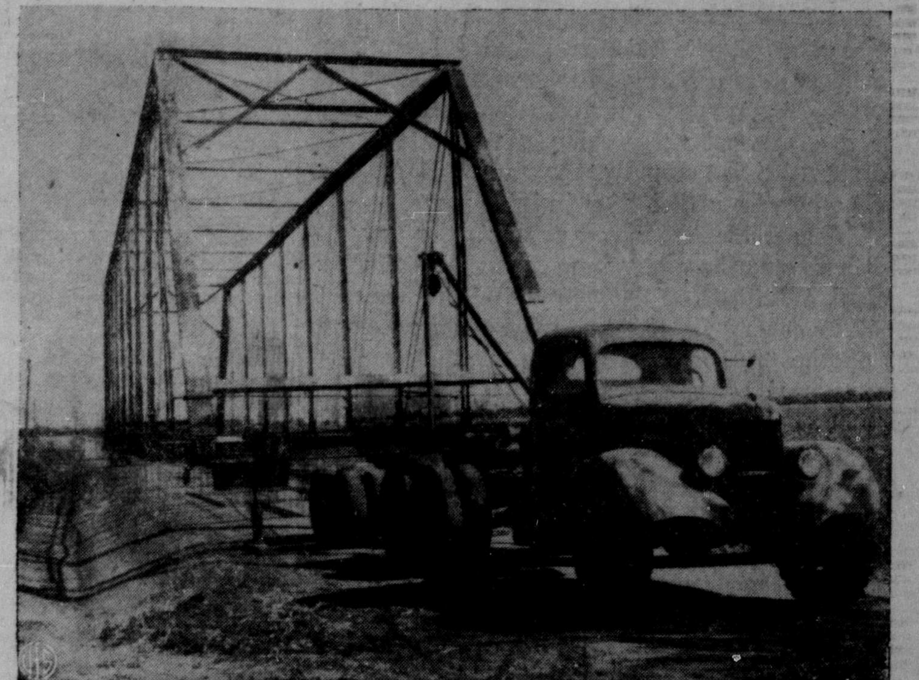
THE SIGHT OF A BRIDGE being towed along the road from Solomon, Kansas, to New Cambria may have surprised local residents, but authorities saw no point in scrapping the big span. It was used to replace one that had been washed away more than 12 years ago, and in its place a brand-new one will be constructed. A house mover provided the equipment needed.
