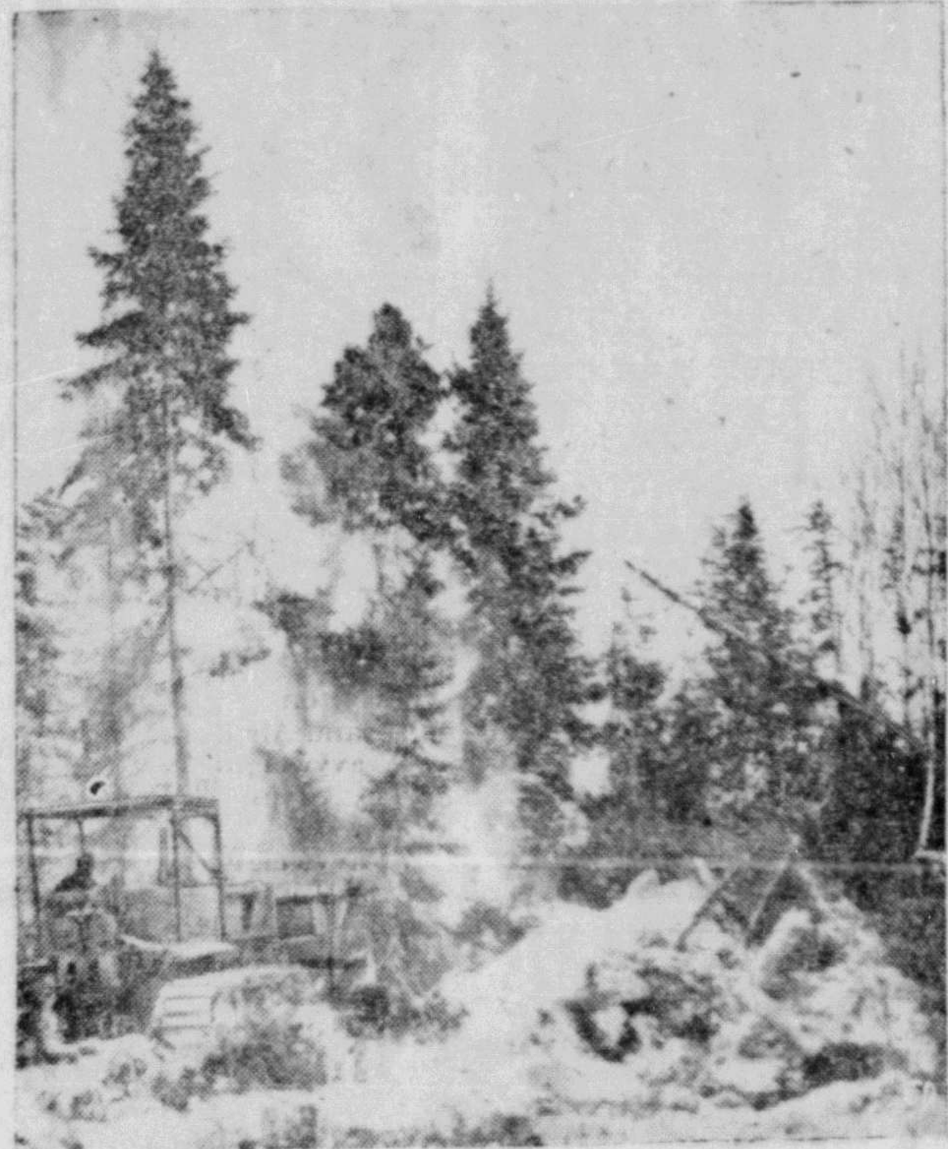
BULLDOZERS PUSH OVER 70-foot trees during the building of the Warren Lake road, running west from Timmins, Ont. The extended road will reach to the Canadian National Railways transcontinental line at Kukatusk.
