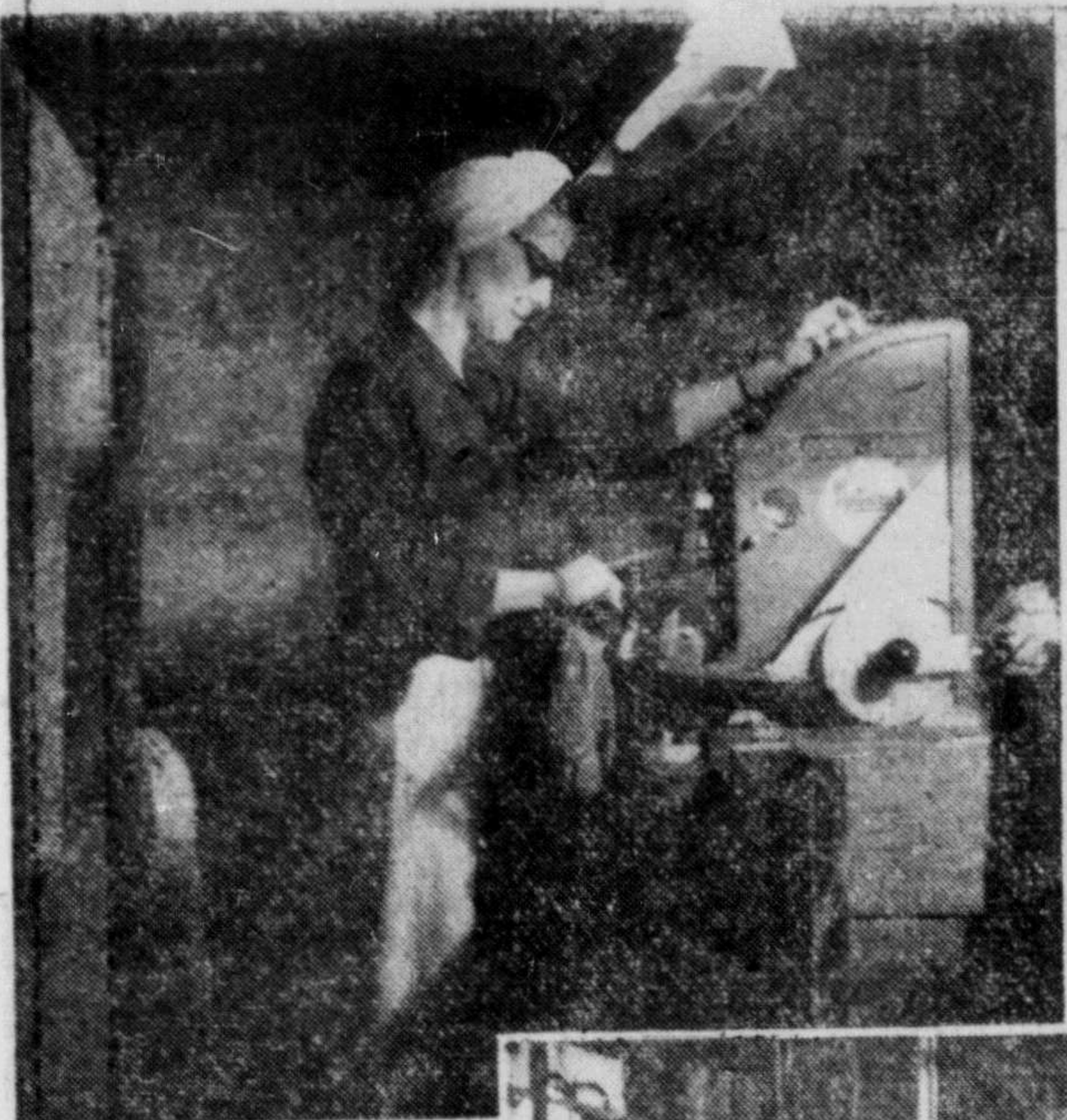
(ABOVE) The new, recently installed "Fantom Fast" visible laundry marking, which is done under ultra-violet light. This invisible marking eliminates entirely all ugly black ink marks previously found as identification on laundry articles.
