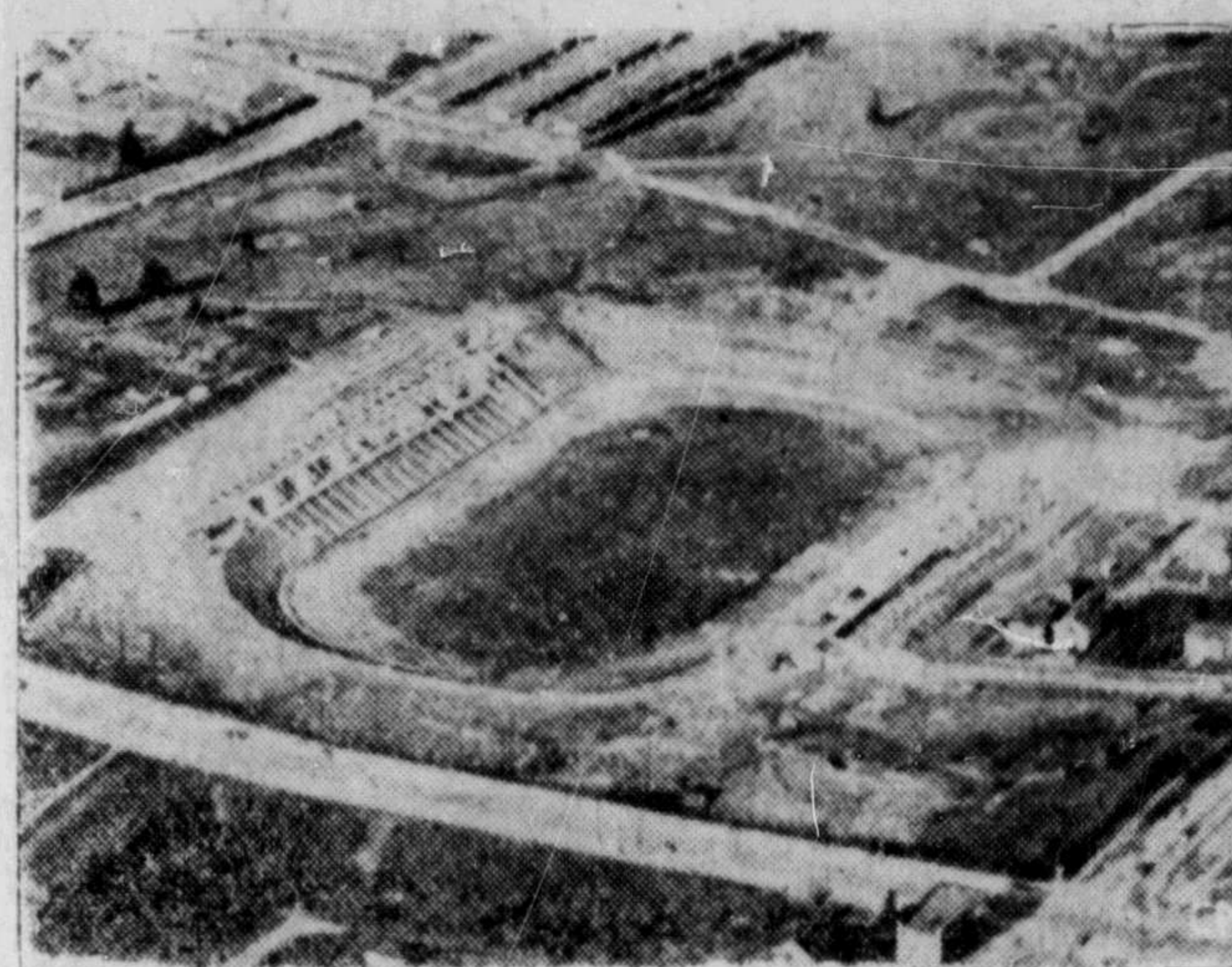
THIS AERIAL VIEW shows construction progress on Canada's largest stadium, to be used for the British Empire Games at Vancouver next summer. To cost $1,895,000 and scheduled for completion April 30, three months before the games start, it will hold 35,000 with 10,000 seats under cover.
