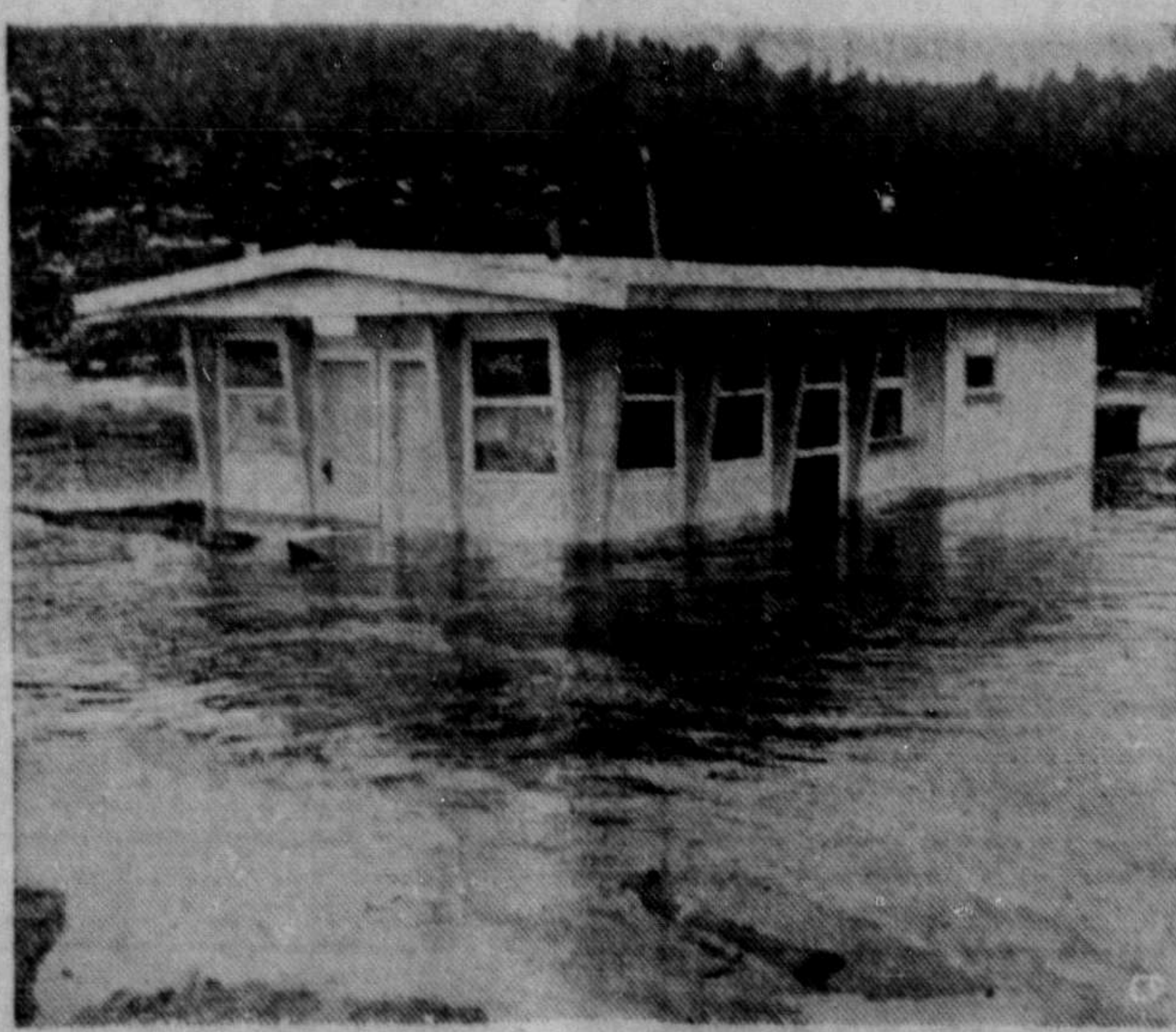
A FEBRUARY RAINSTORM, termed "phenomenal" by weather experts, washed out bridges, railway tracks, caused temporary evacuation of 25 families and marooned dozens of families in Nova Scotia. This is what happened to a snack bar near Halifax.
