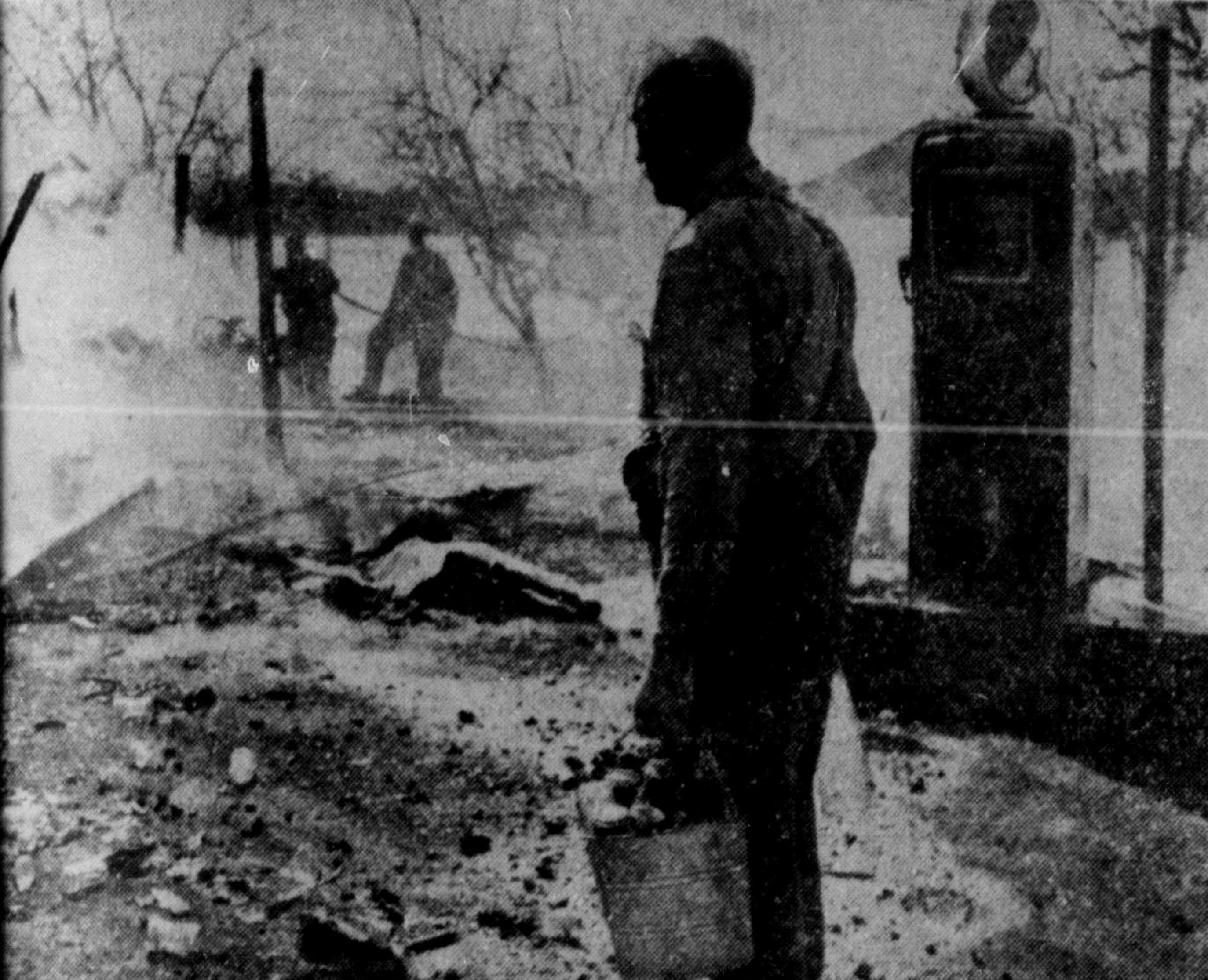
Fire Destroys Garage
