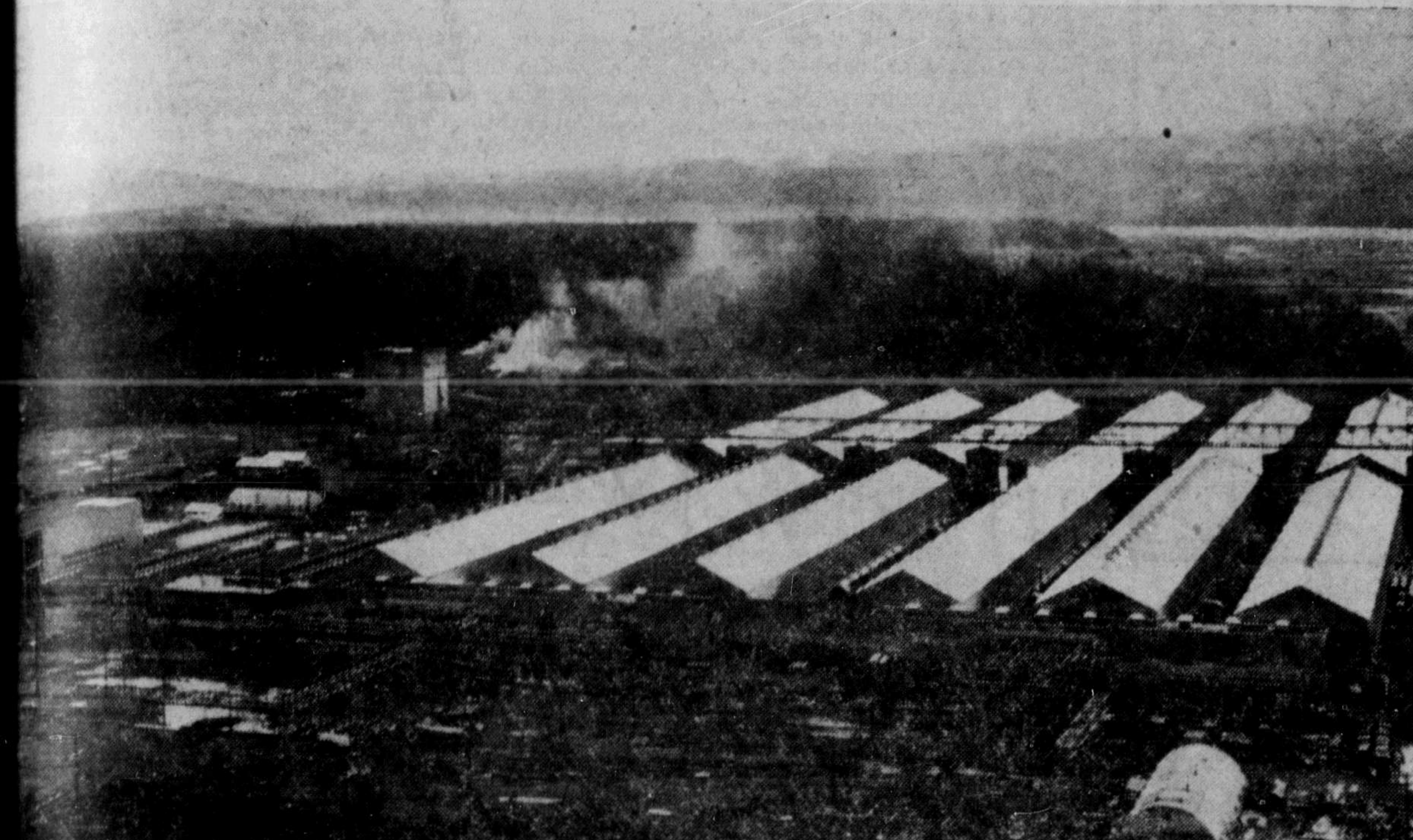
BEST PICTURE of the giant Aluminum Company of Canada plant at Kitimat shows the main plant, seven miles from Kitimat townsite. Six peaked buildings dominating the scene are the completed pot lines where actual production of aluminum is carried out. Alumina will be stored in huge sheds (not shown) and brought in on overhead conveyor, centre. A paste plant, already in operation, is shown at extreme left.
