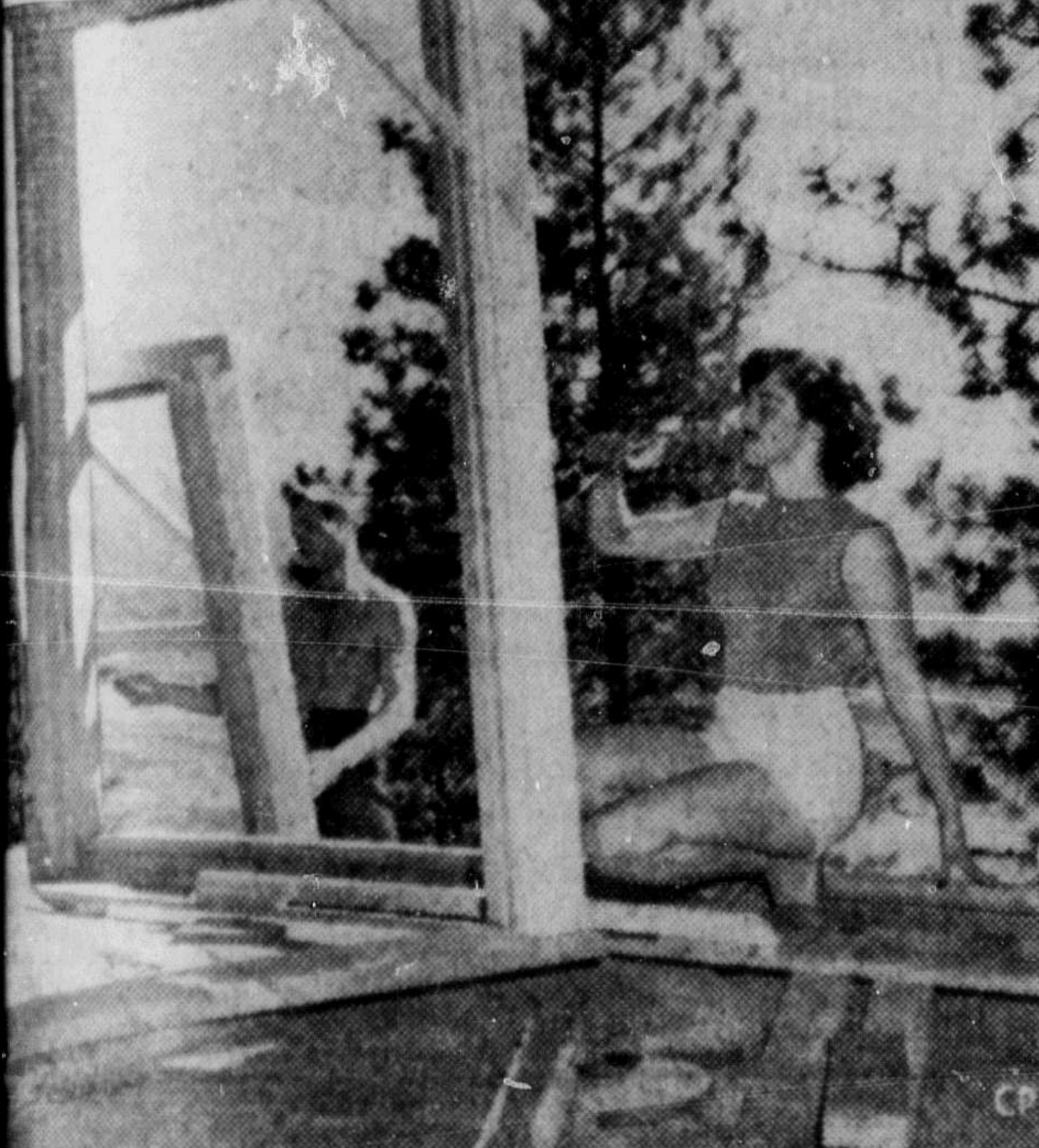
PLYING THE PAINT—From Kamloops in the north of British Columbia down through the Okanagan Valley to Keremeos near the United States border, six separate joint Prairie Farm Rehabilitation Administration and Veterans' Land Act irrigation projects are under way. Qualified ex-servicemen are busy turning wilderness into production acreage. The largest project is Westbank, across the Okanagan Lake from Kelowna. Mr. and Mrs. George Stevenson, full-time farmers of the Westbank project, are applying a priming coat of paint to a window sash on their home. (CP from National Film Board)
