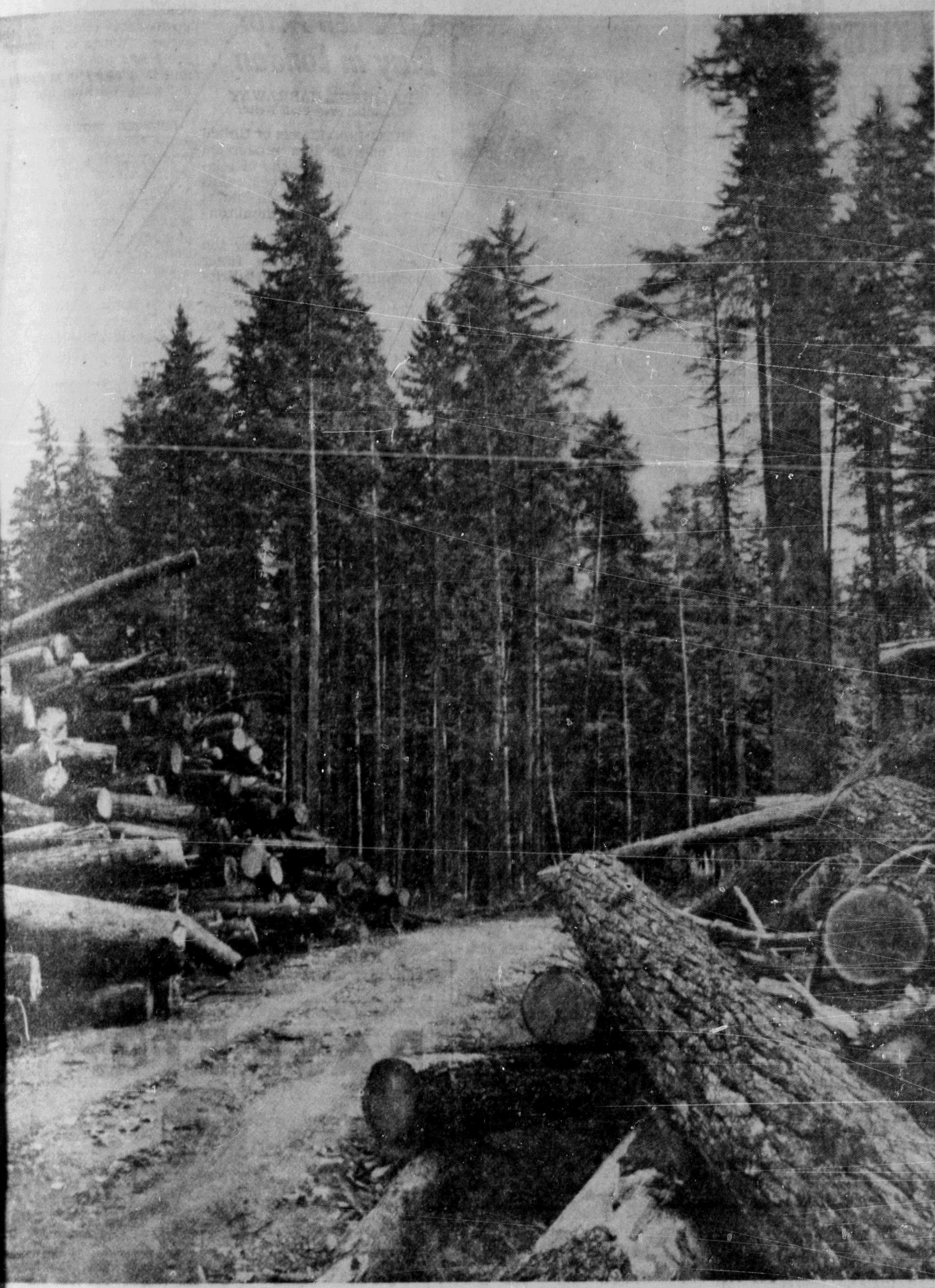
LOADING LOGS AT TERRACE—Woods scene in Kitsumkalum area at Terrace which is producing millions of feet monthly.
