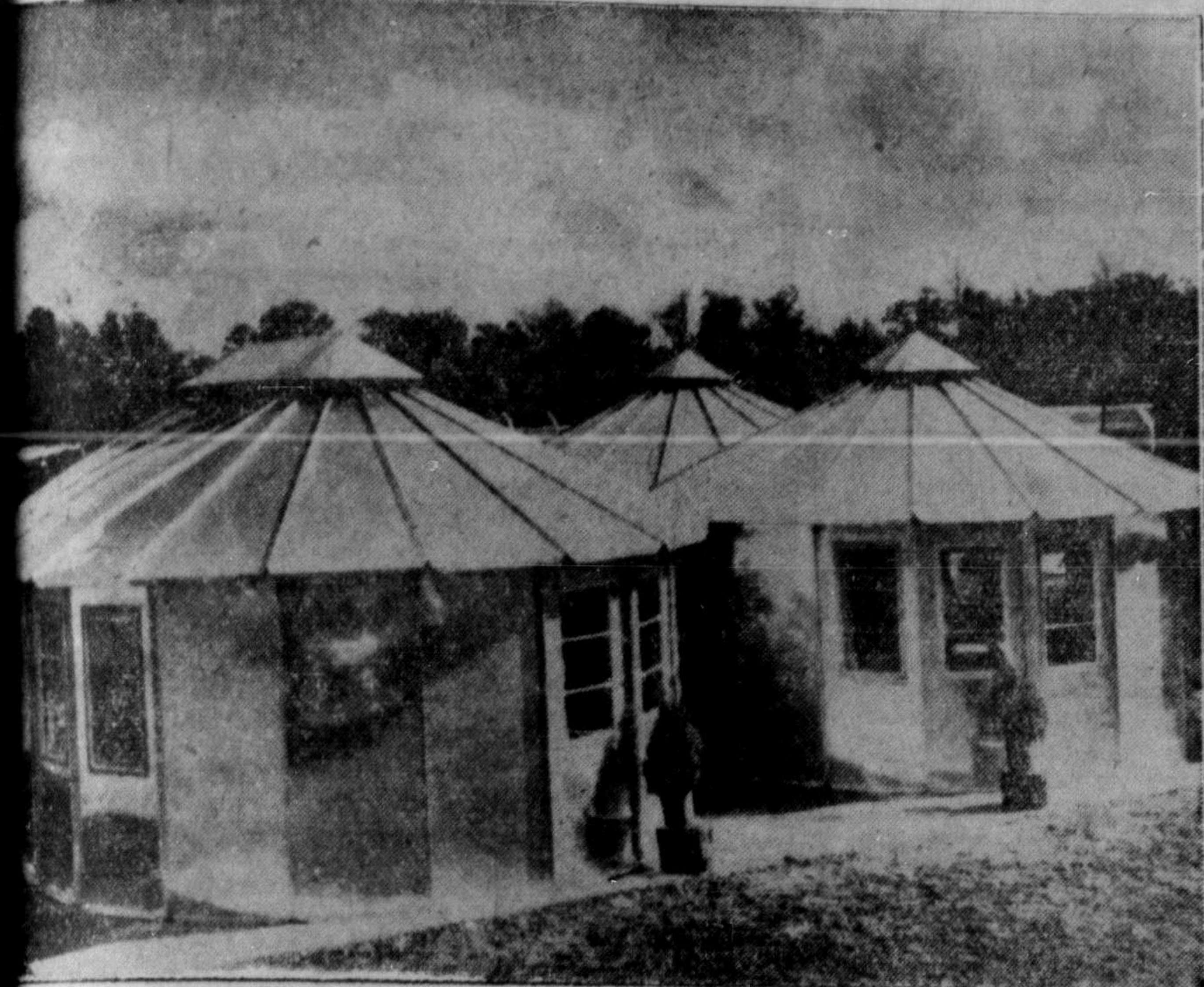
PORTABLE ALUMINUM "PALACE" is being exported by a British firm to the Persian Gulf for use as a hunting lodge by Crown Prince Saud of Saudi Arabia. The construction consists of a group of prefabricated buildings, each of which can be erected or dismantled in an hour and transported in sections by camel.
