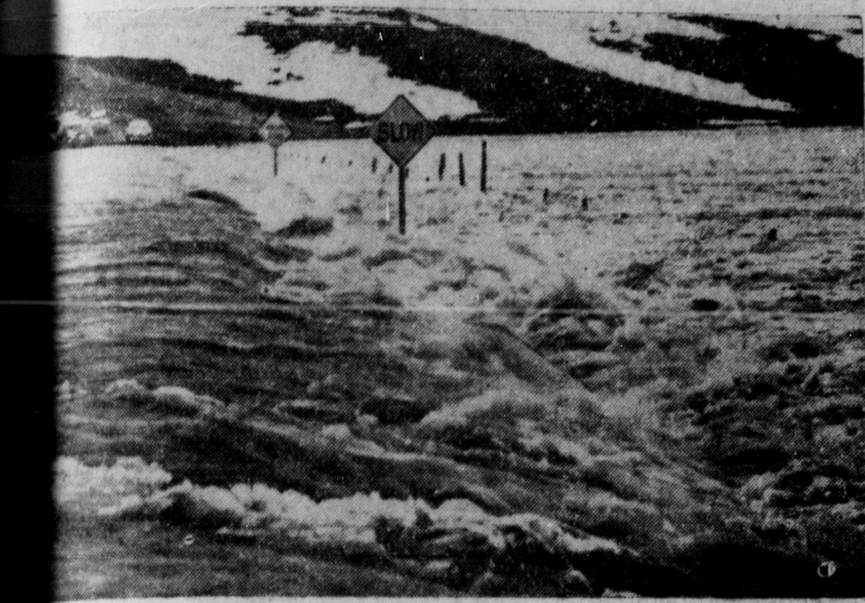
FLOODED—Flood conditions in some parts of western Canada have been severe and caused heavy damage. This is a view of Saskatchewan's No. 4 highway where the Eagle Creek, north of Rosetown. Water—now subsided—was at least a foot deep for 300 yards. (CP PHOTO)
