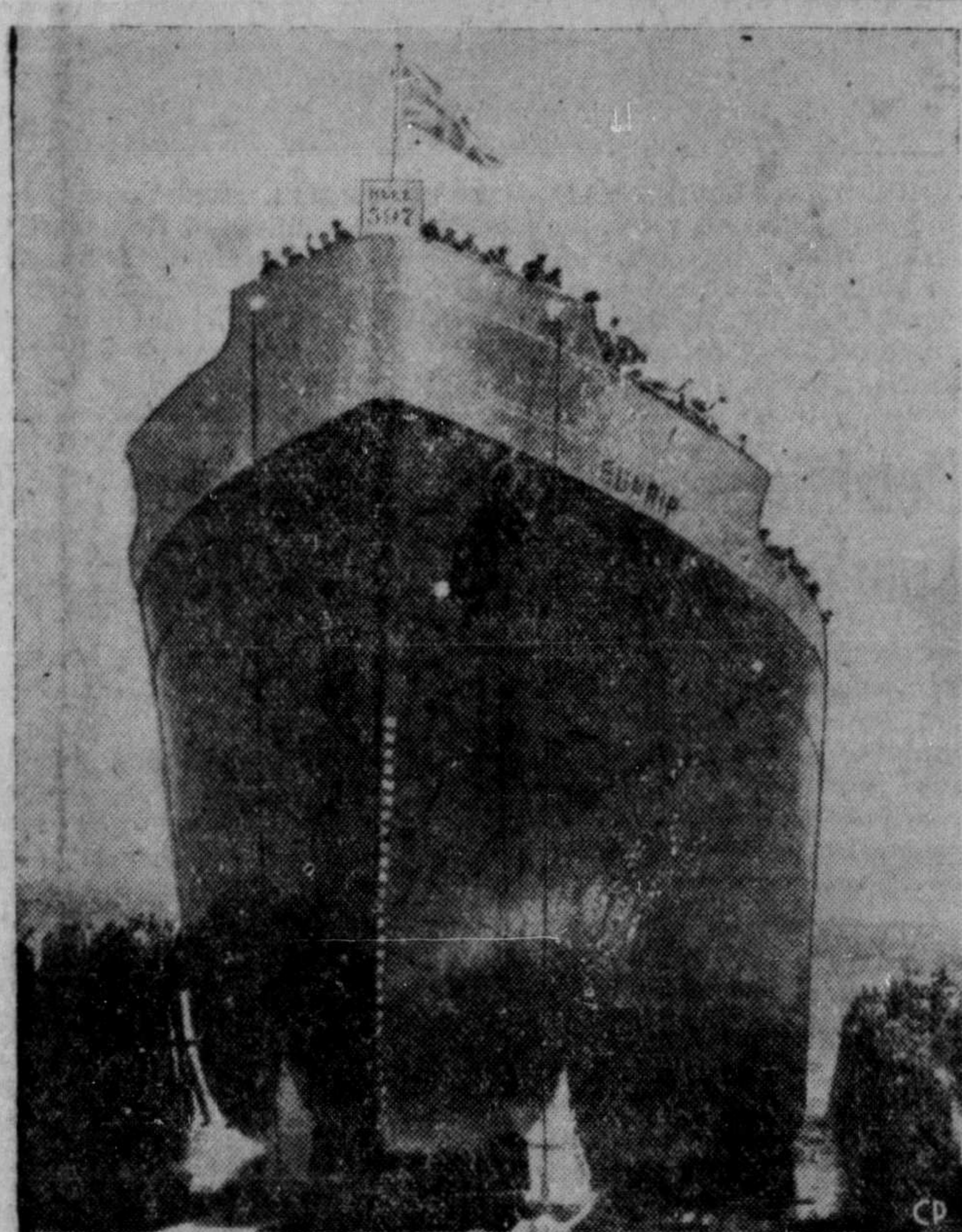
THE 12,400-TON SUNRIP , largest ocean-going freighter ever built in Canada, slides down the ways at Lauzon, Que. Built by Davie Shipbuilding and Repair Company, the 475-foot vessel will carry bulk aluminum oxide from Jamaica to the Alcan smelter at Kitimat, B.C. The freighter is the first major merchant vessel to be built with an all-welded aluminum superstructure and is designed to maintain a service speed of 13½ knots. (CP Photo)
